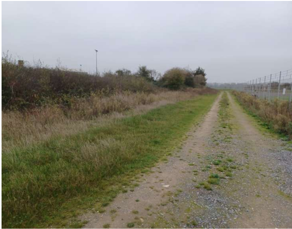
View of the new access road location in the north
