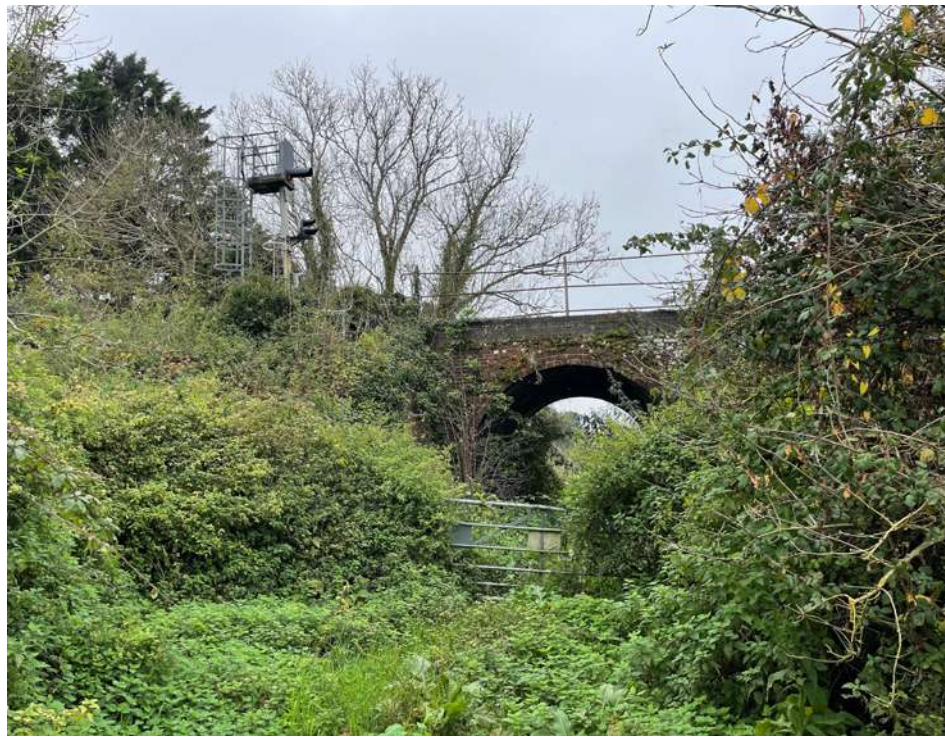
View of the Chicken Hall Lane access
