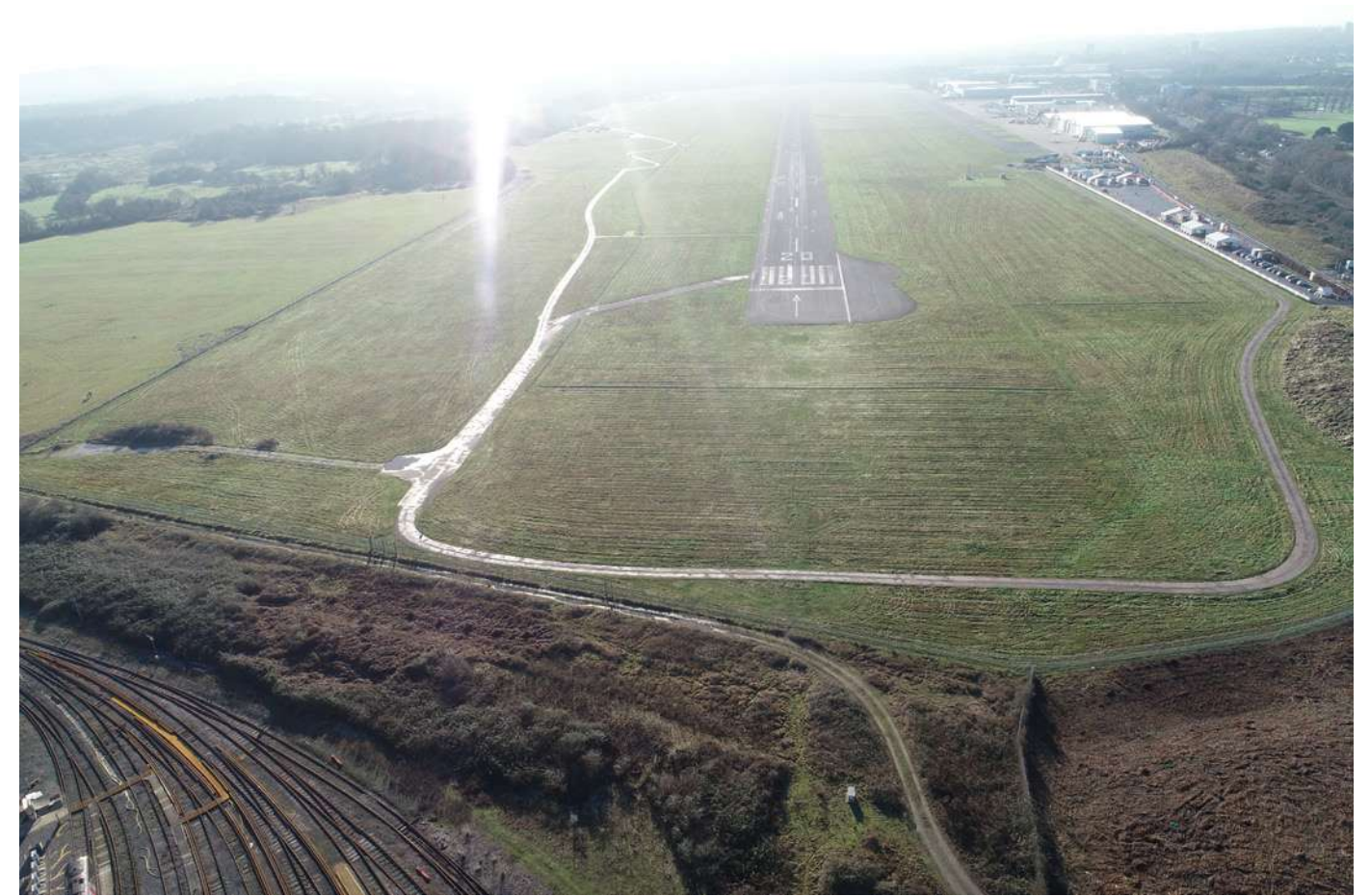
View of the Airport runway from the north boundary
