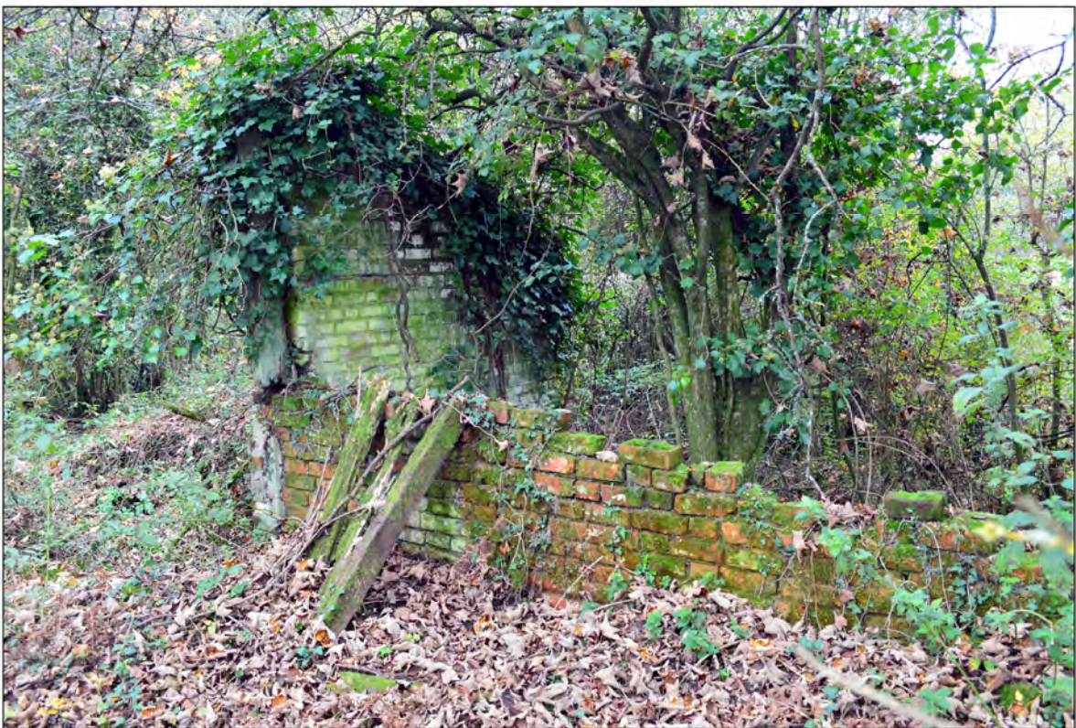
Photo 8) Structural remains of North Stoneham Farm at the southern edge of Plot 2
