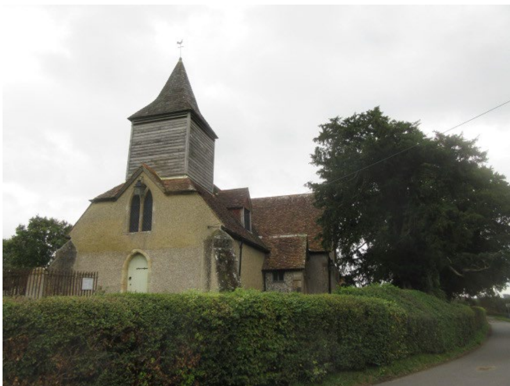
Plate 1: Church of the Holy Cross, looking east
