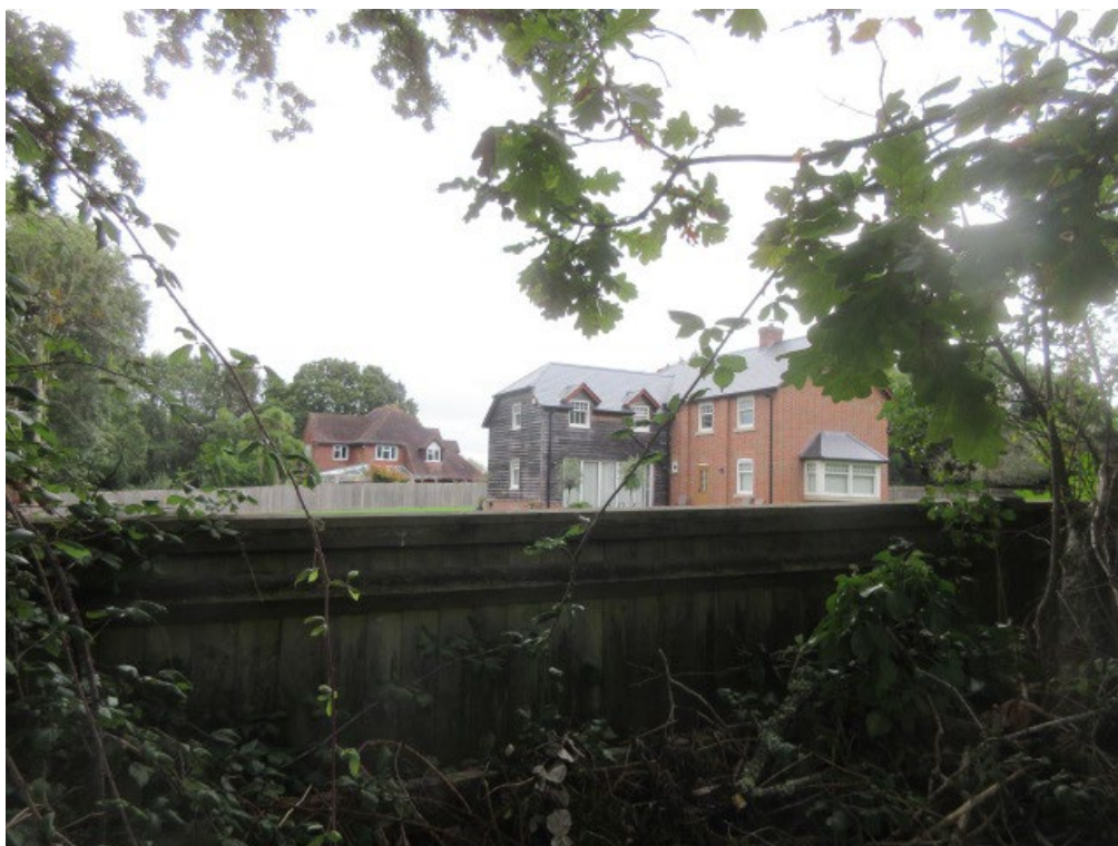
Plate 6: Buildings at Lane End Farm, looking north
