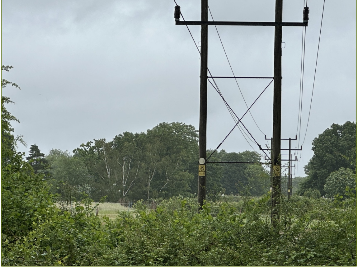
Figure 2 – View from bridleway (public right of way )026/17/2 looking north
