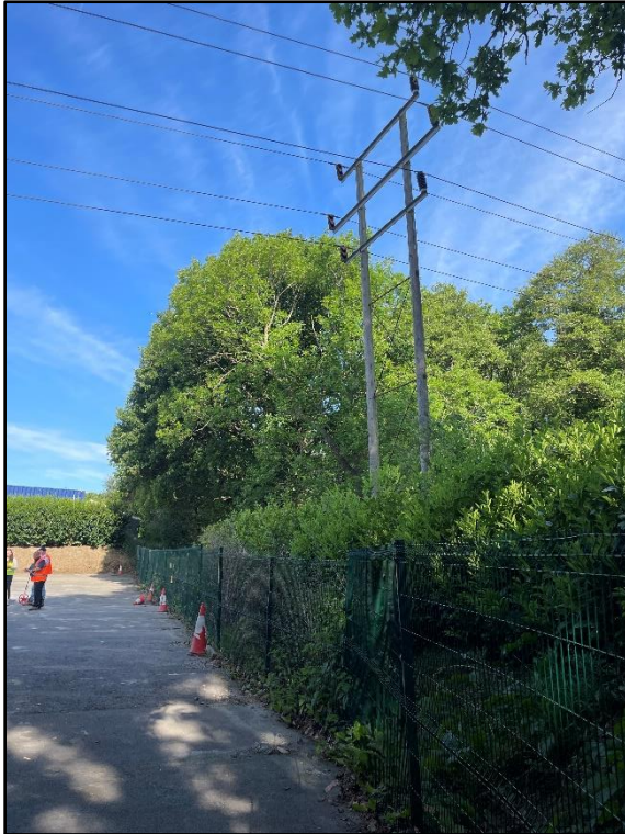
Image 5: View of northern perimeter from eastern vantage point highlighting the location of electrical power services.
