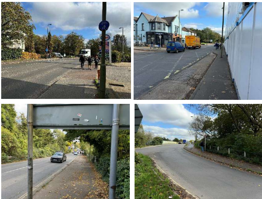
Figure 6-5: Site Visit Photos – Route 2, Section C
