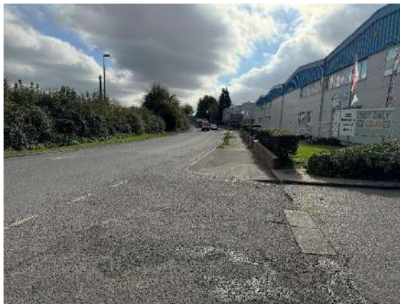
Figure 6-4: Site Visit Photos - Route 2, Section B
