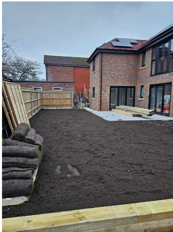
Photograph 9: Dwelling completed and rear gardens surfaced with topsoil
