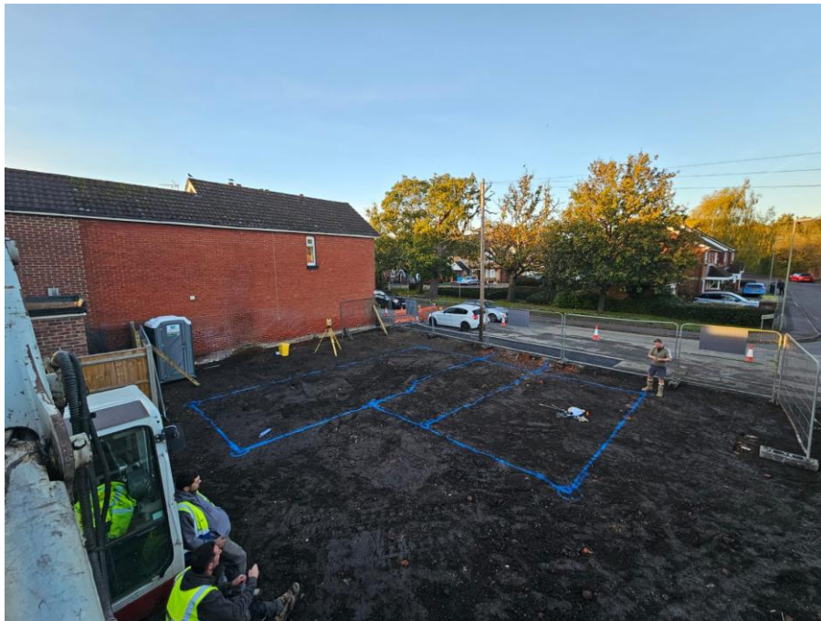
Photograph 1: Site area cleared and foundations marked out.
