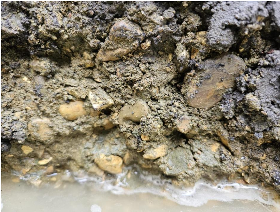
Photograph 7: Gravels within clayey sands. Water within the trench.
