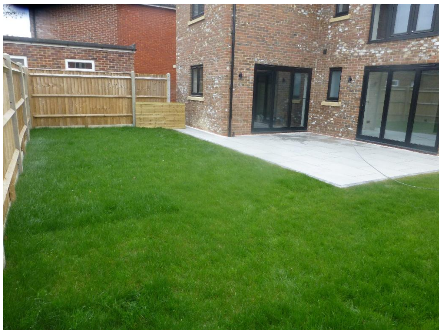
Photograph 12: Completed rear turf at the site.
