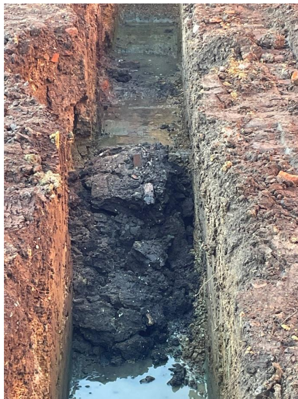
Photograph 4: Continuation of digging of the foundations
