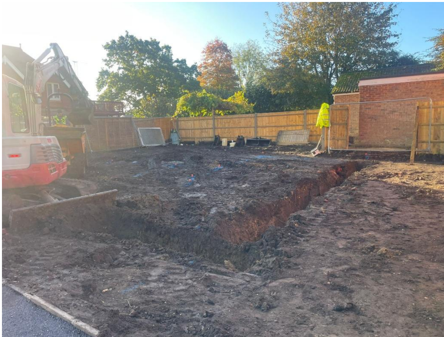
Photograph 3: Continuation of digging of the foundations
