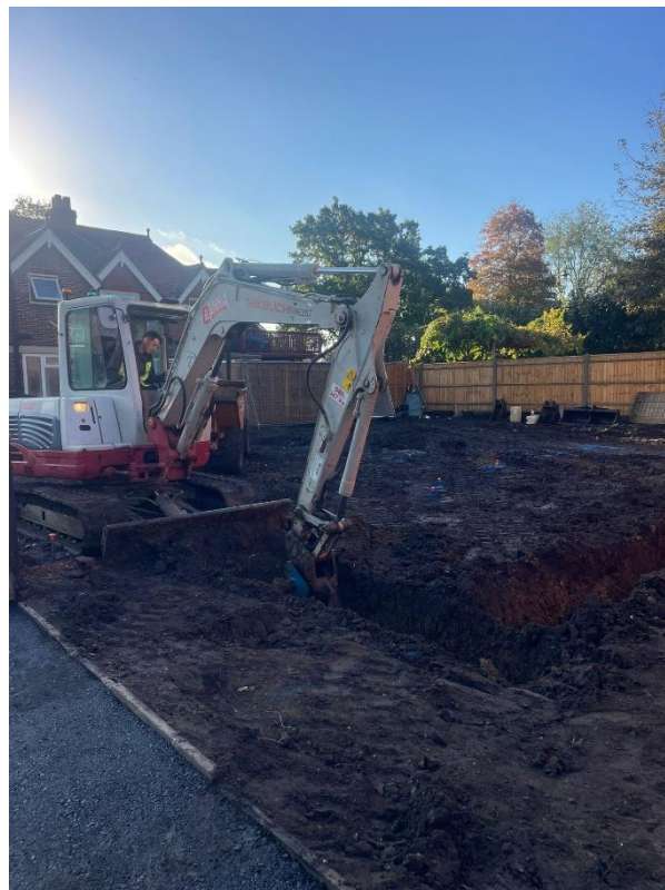
Photograph 2: Digging of the foundations
