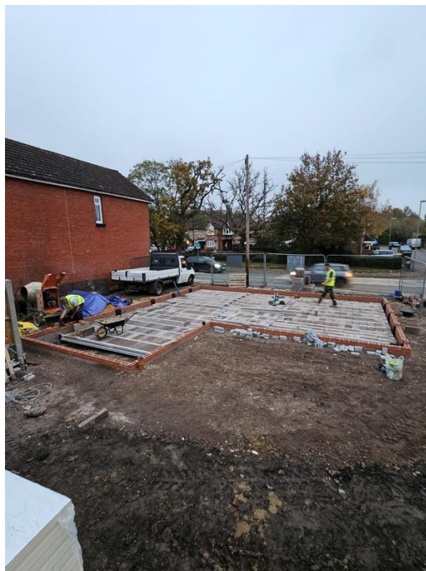
Photograph 8: Foundations completed to ground level.
