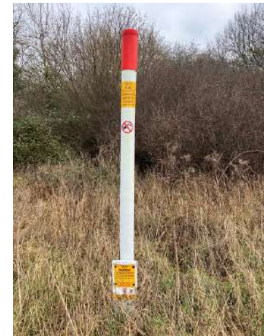
Image 6: High pressure gas main marker along northeastern boundary
