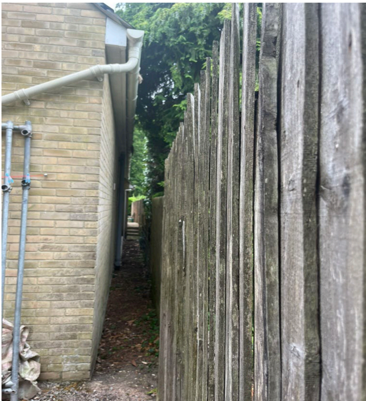
Fig.2 – Photograph showing the West elevation on which the flue is to be situated showing fence line with neighbour to right hand side
