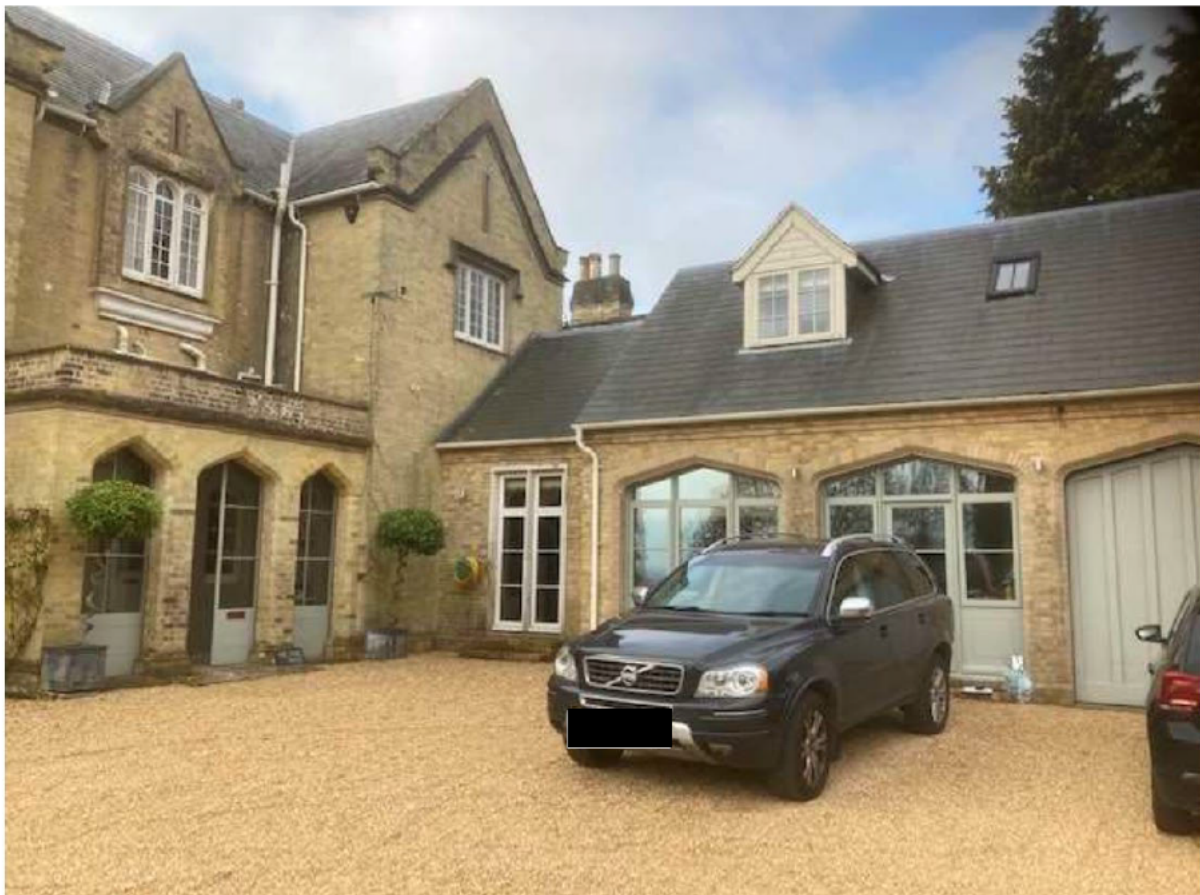
Fig.1 – Photograph of Hoe Moor House East facing elevation with main entrance on left hand side.
