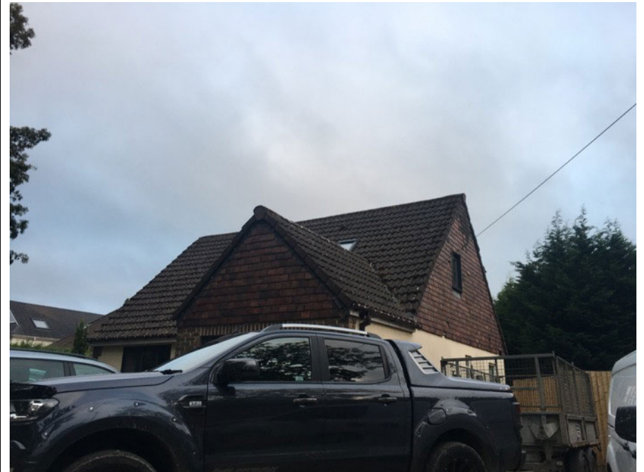
North-eastern corner view from NVA at start of survey. Unfortunately the end still was lost at this location due to a corrupted SD card.
