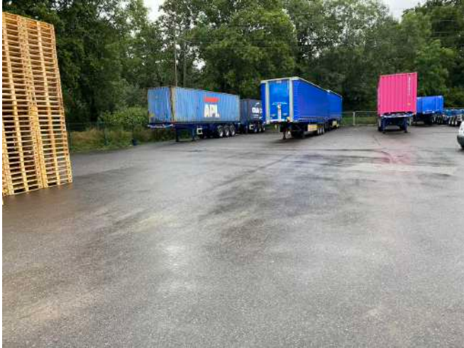
Plate 5: Parcel G7 hardstanding (grasscrete prior to 2021)
