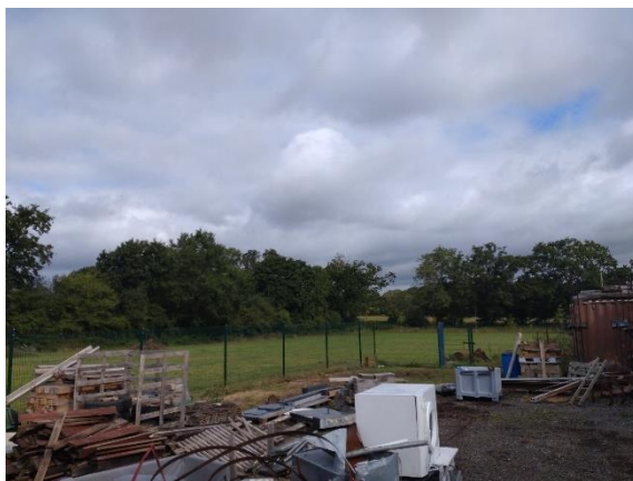
Photograph 2: Existing conditions at site of new parking area
