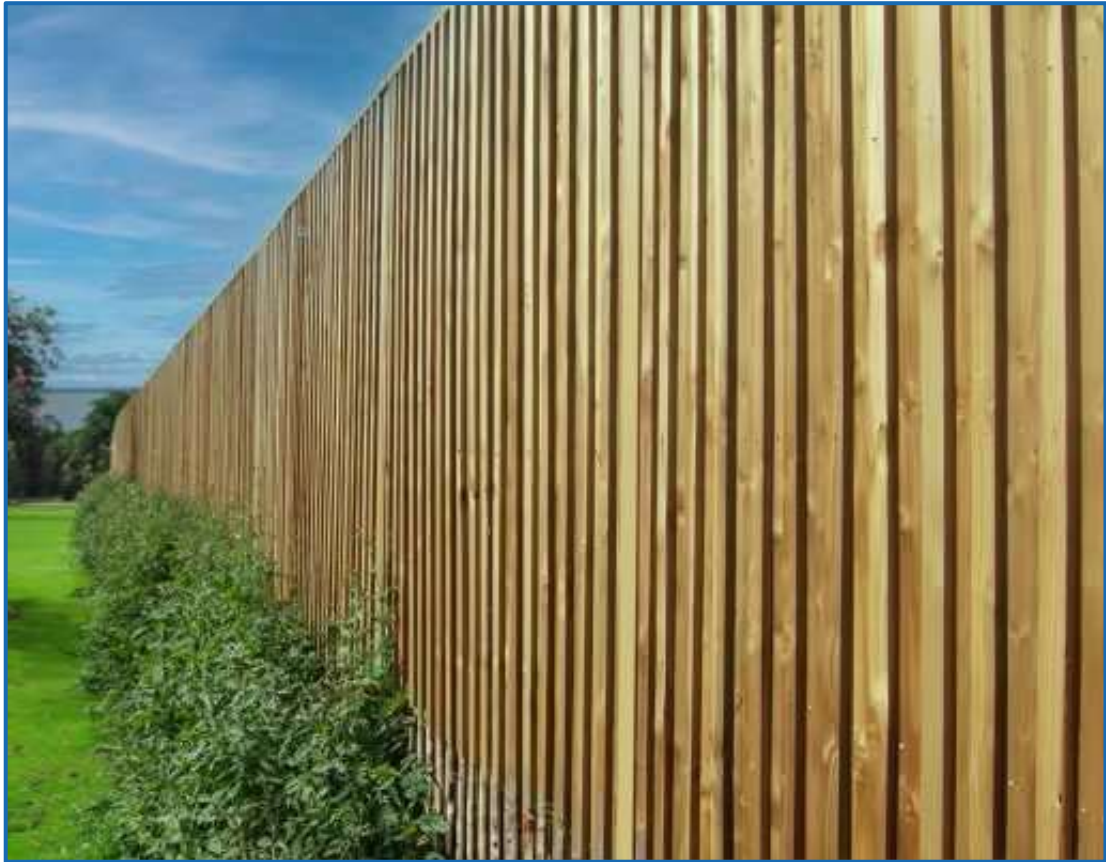
Figure 2: Example of a Solid Boarding Fence 6
