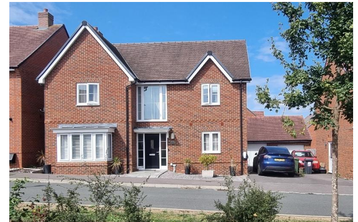
Front façade face East towards Lewry Road.
