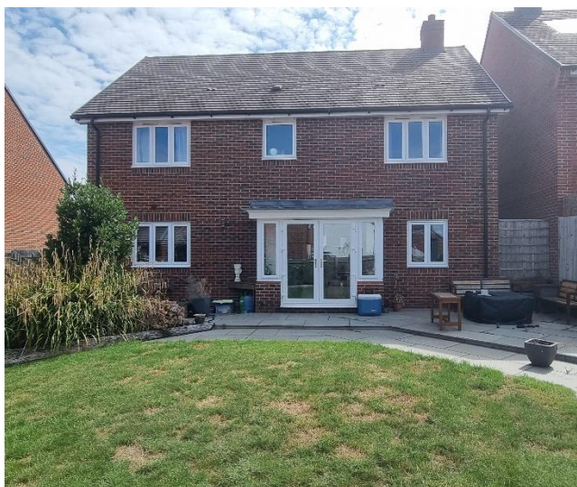
Rear garden West facing elevation.
