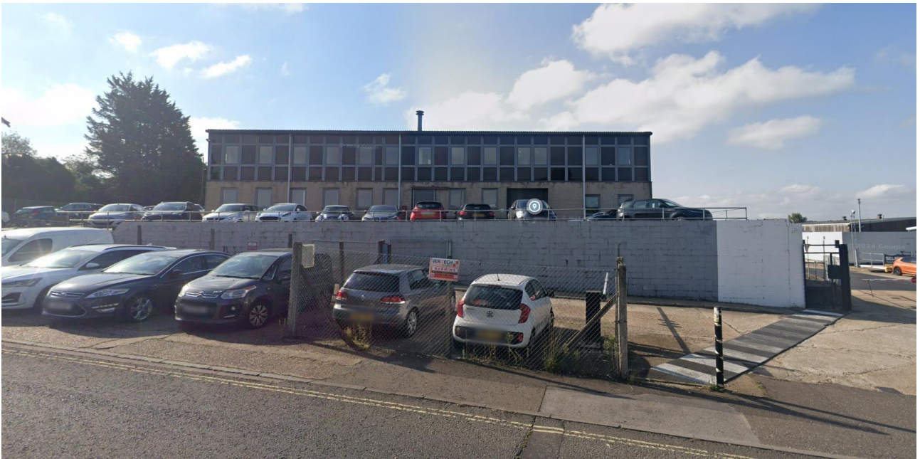
Figure 16. View from north side of site looking up the terraces towards the existing headquarters building, showing the retaining wall and terracing of the site (Google Maps Accessed 17/06/2025).
