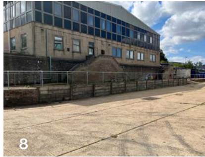
8 West (back) elevation of existing office HQ
