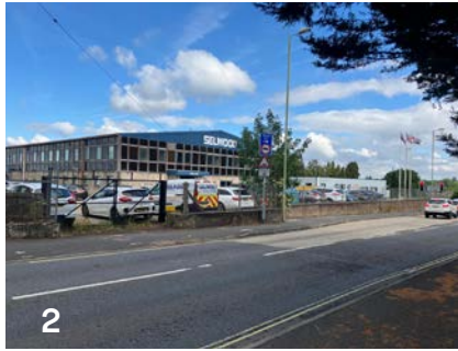
2 Bournemouth Road frontage block
