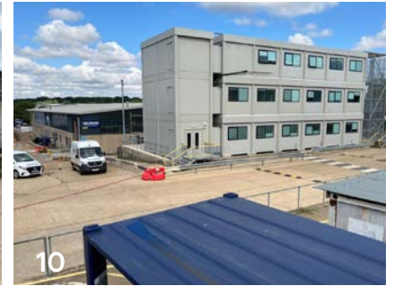
10 Temporary office building
