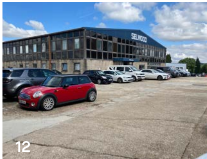
12 Hardstanding in front of existing office HQ
