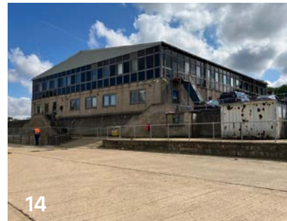
14 Existing office HQ and access driveway
