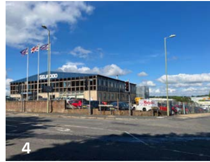
4 Bournemouth Road / School Lane junction
