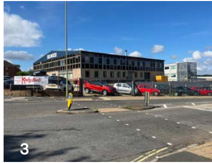
3 Existing Office HQ
