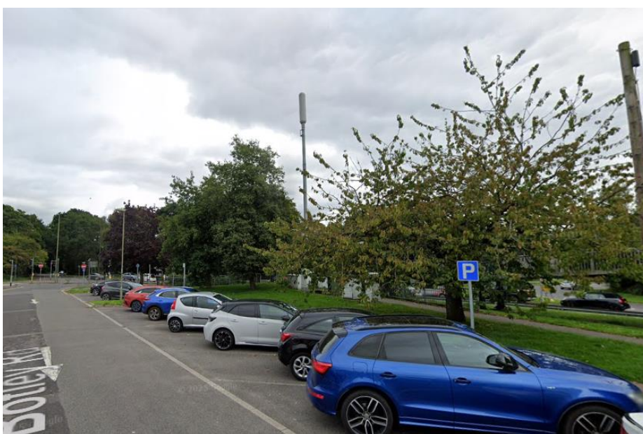
Figure 2 – Botley Road Mast (not considered/approached for site sharing) despite close proximity to search area.
