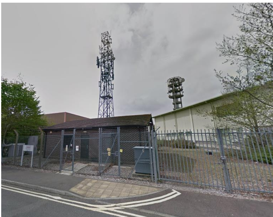
Figure 1 – Image of mast (foreground) not considered for site sharing despite close proximity to search area. Existing mast in background.
