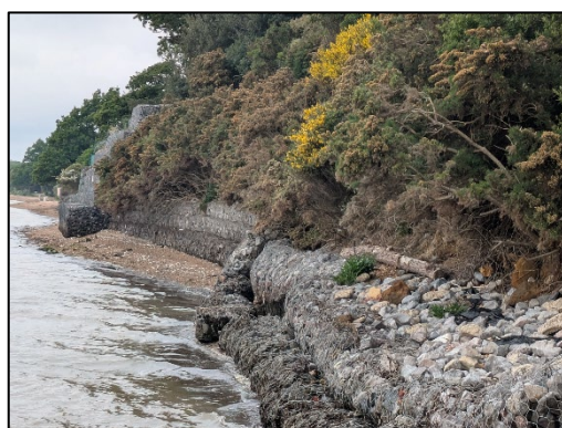
Figure 2: View of the retaining wall meeting the beach front.
