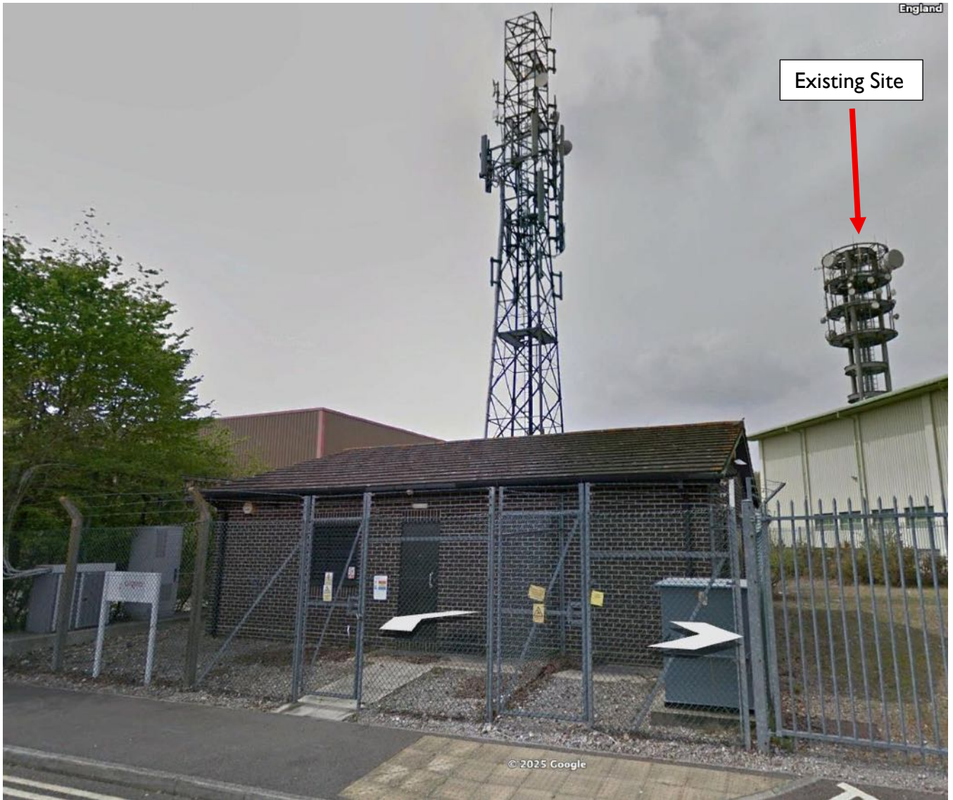
Existing site (red arrow) taken from Manaton Way
