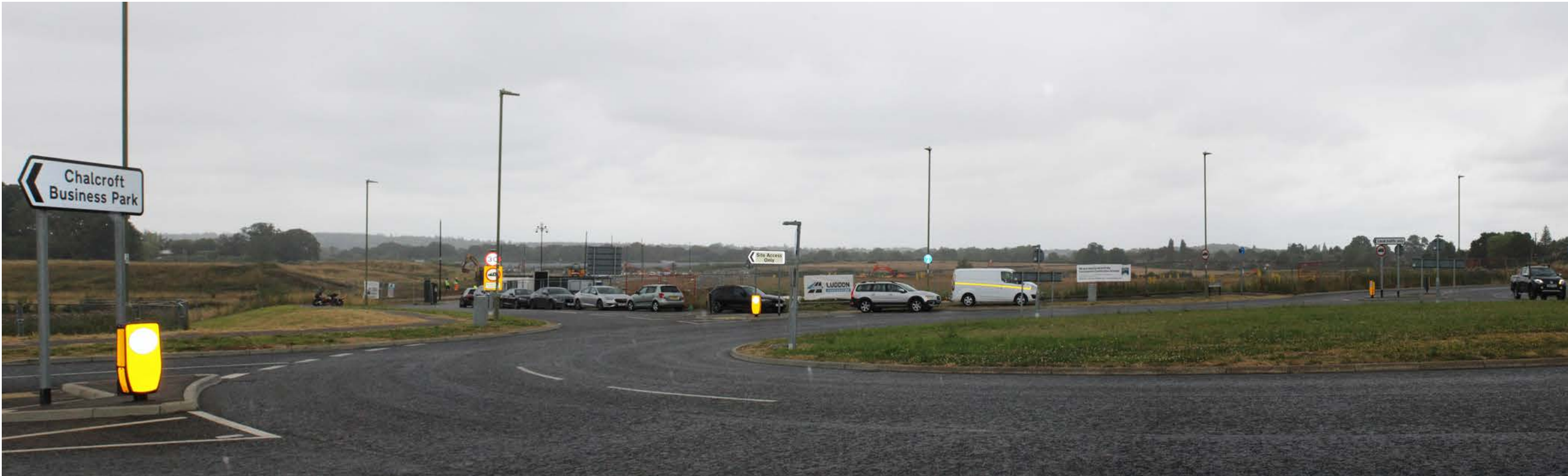
Updated Photoviewpoint 14 (July 2024): The view is dominated by the Bubba Lane/Burnetts Lane roundabout and construction activity associated with Phase 1
