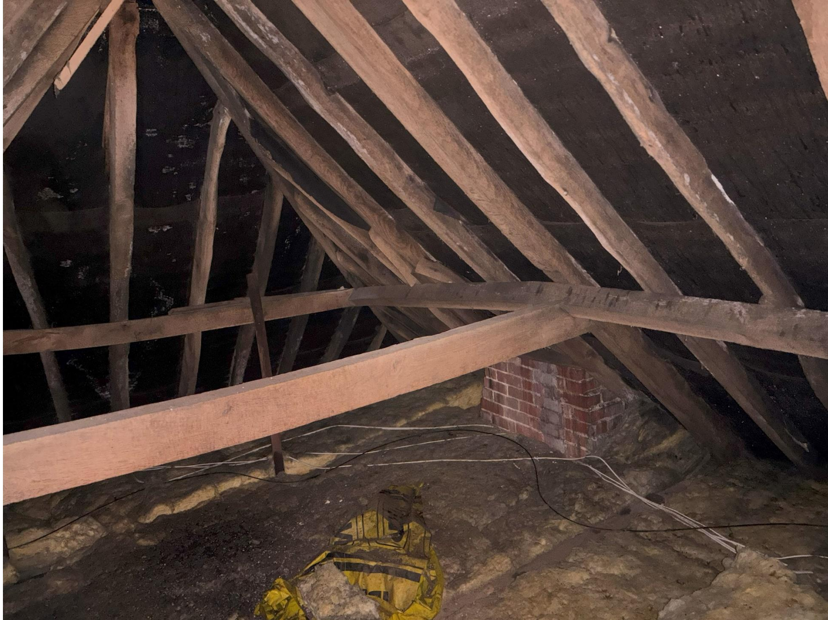
Stroudwood Farmhouse – Roof Repairs – Listed Building Application
