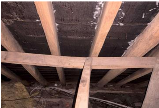
Fig. 16: A deflecting purlin joint.
