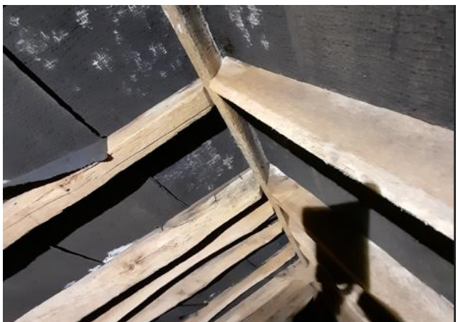
Fig. 19: Widening joints between rafters and ridge-beam.
