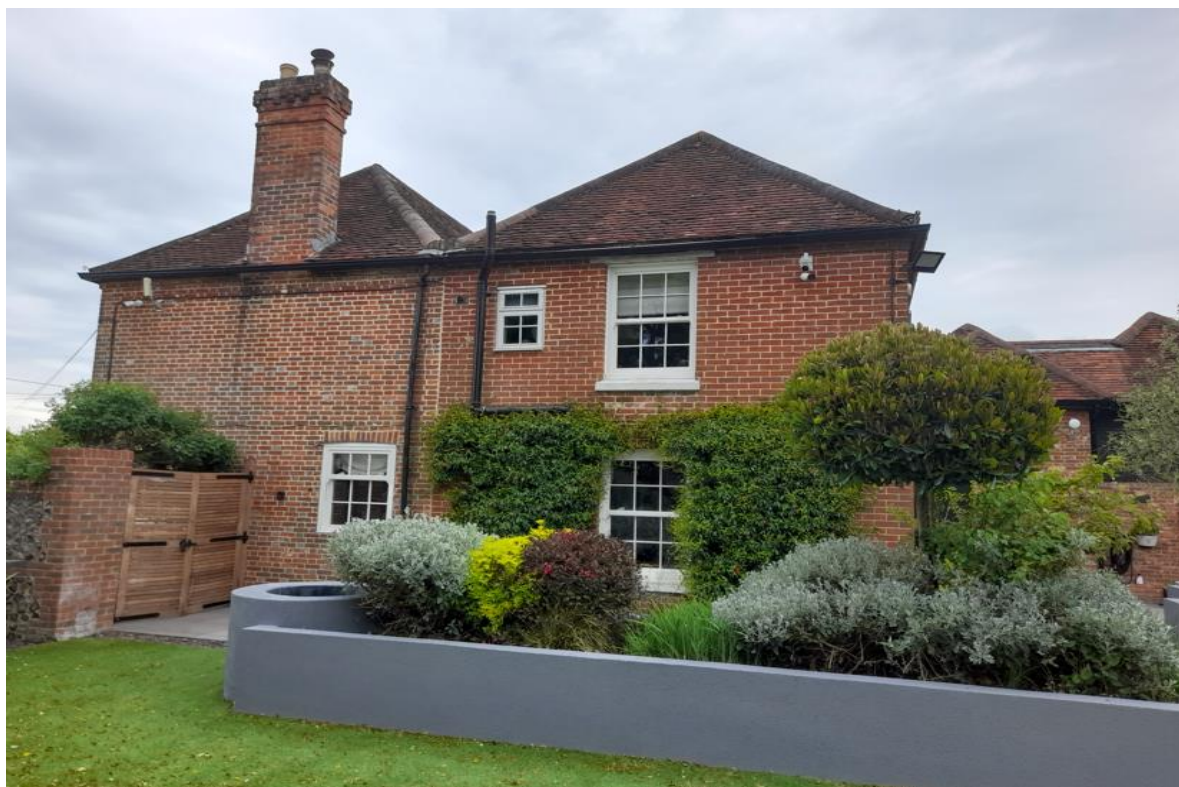
Fig. 6: View, looking south-west of the east elevation of Stroudwood Farmhouse, with double-span hipped roof and two distinct phases of brickwork construction.
