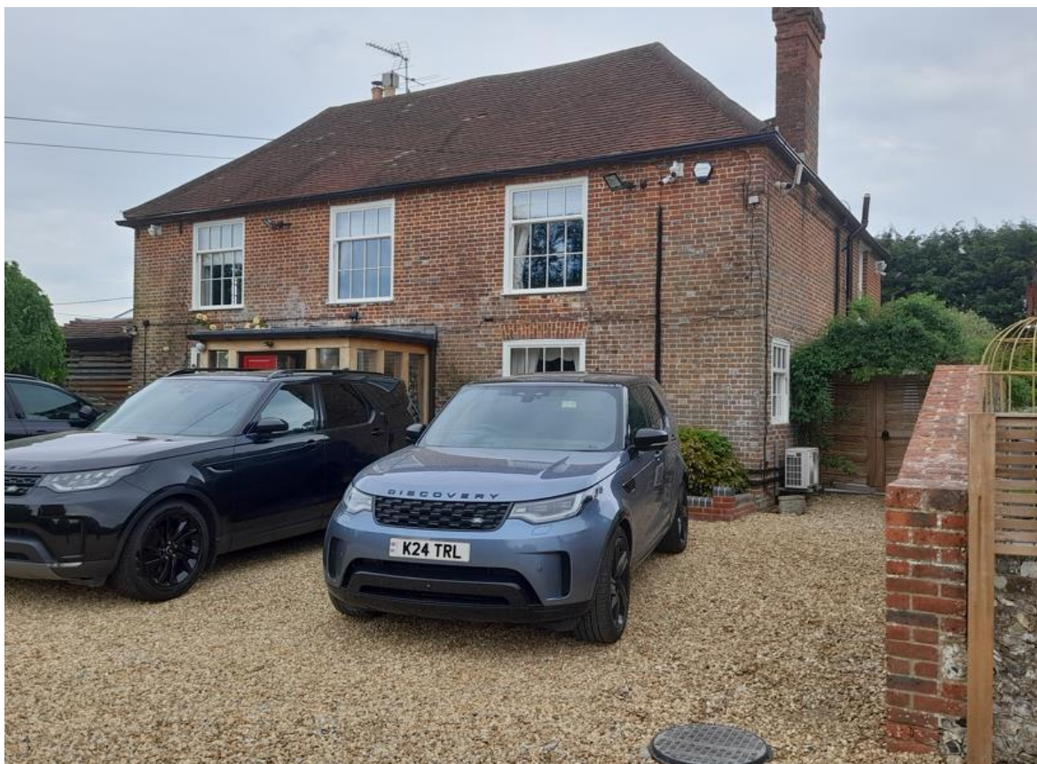
Fig. 5: View, looking north-west, of the south and east elevations of Stroudwood Farmhouse.
