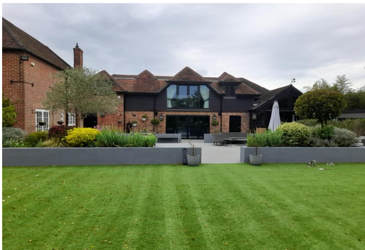
Fig 7: View looking east, of the north elevation of Stroudwood Farmhouse and surrounding garden and adjoining converted barn.
