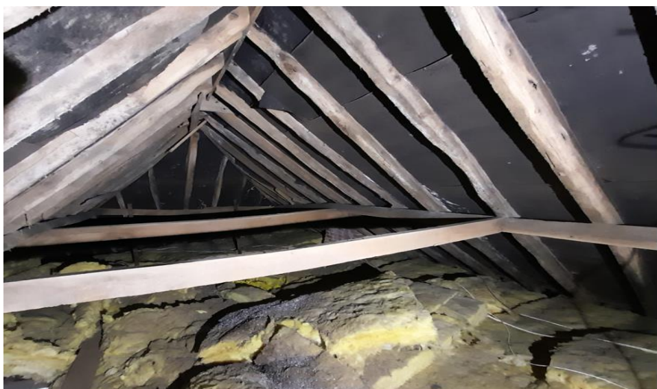
Fig. 8: View, looking west within the roof-space, with details of timber-framed construction.
