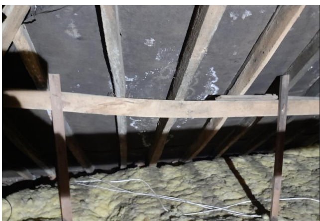
Fig. 17: A purlin supported off ceiling joists.
