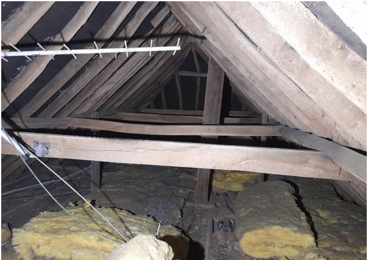
Fig. 12: View looking east within the affected roof-space, with detail of timber construction.
