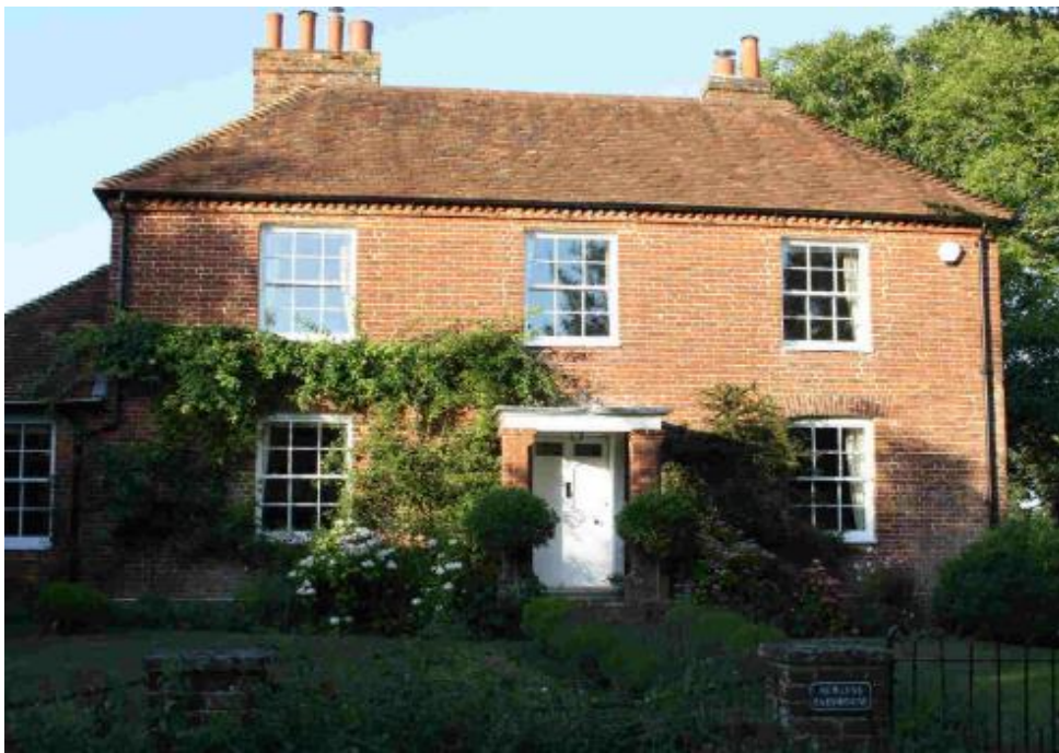
Fig. 4: The south, front elevation of Stroudwood Farmhouse.
