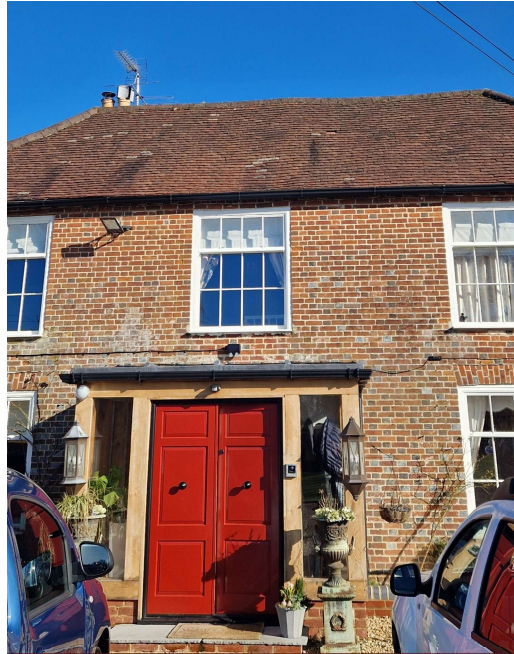
Figure 1 – Front (South) elevation of Stroudwood Farmhouse
