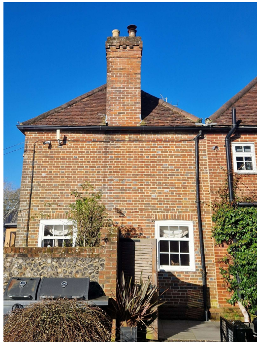
Figure 2 – Side (East) elevation of Stroudwood Farmhouse
