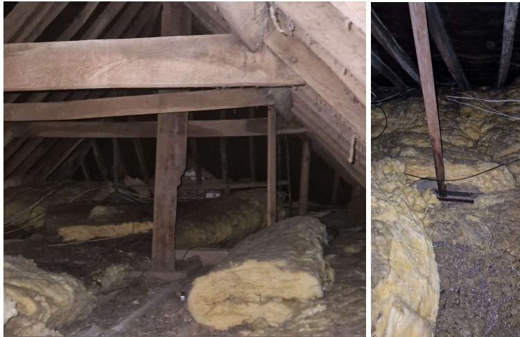
Figures 7 & 8 – Purlins supported off ceiling joists
