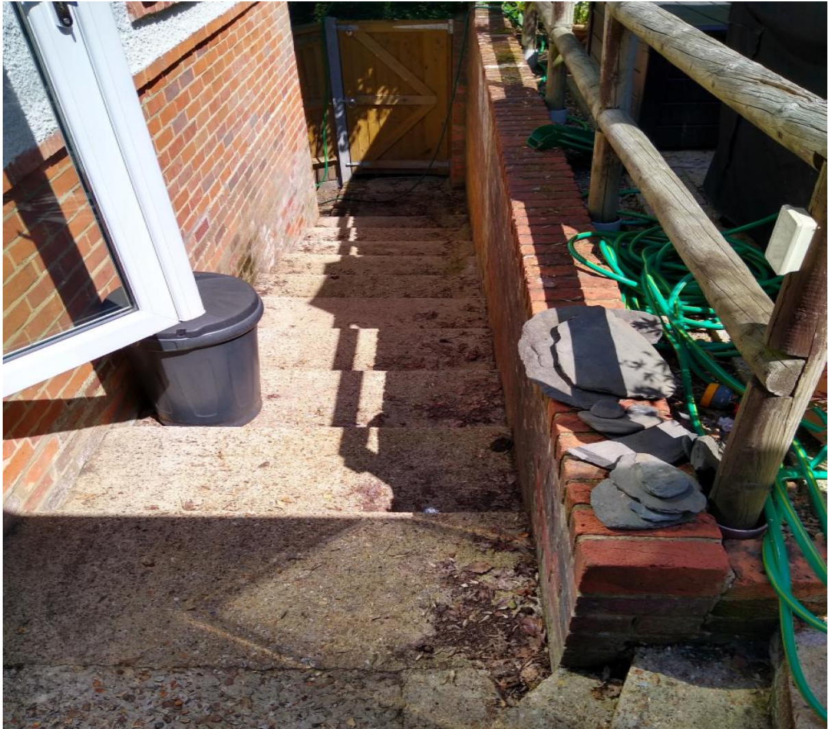
Image 6. Showing the steps running across the back of the living room and study. Note the awkward height of the bottom of the patio door shown to the left above the ground level at that point.
