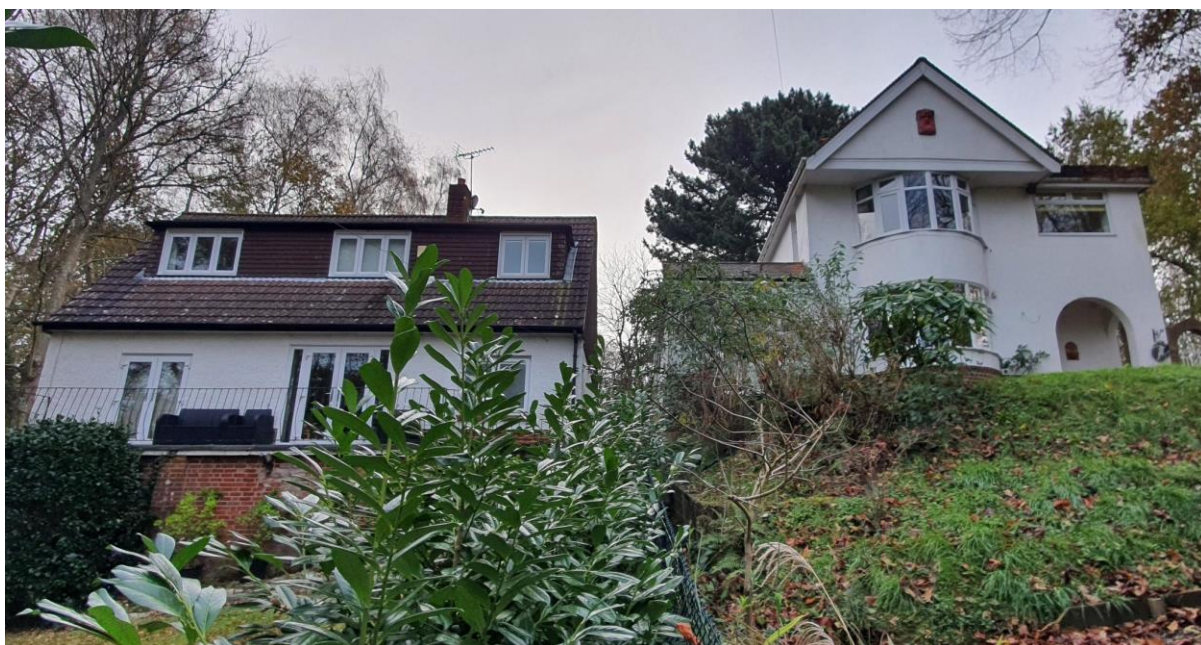
Image 3. St Georges and Longwood as viewed from the driveway on the boundary of the two properties.
