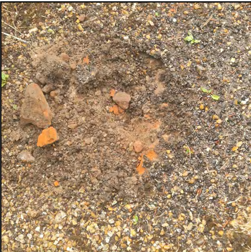
Photograph Five – Gravel/hardcore drive
