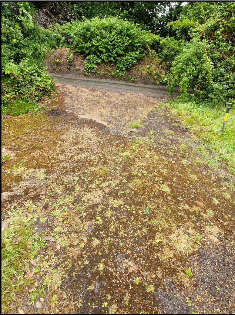
Photograph Four – Concrete apron with gravel to right
