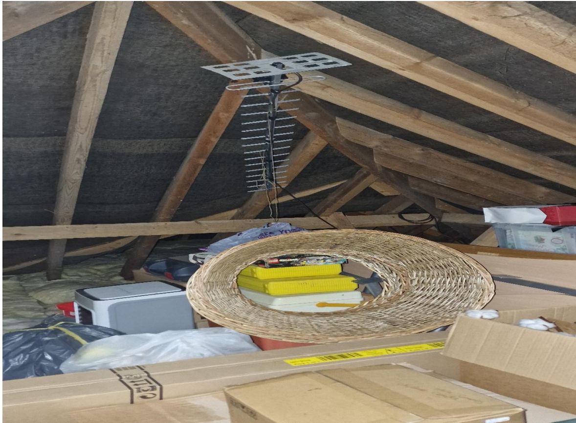
Picture 6: Showing the internal roof structure of the house.
