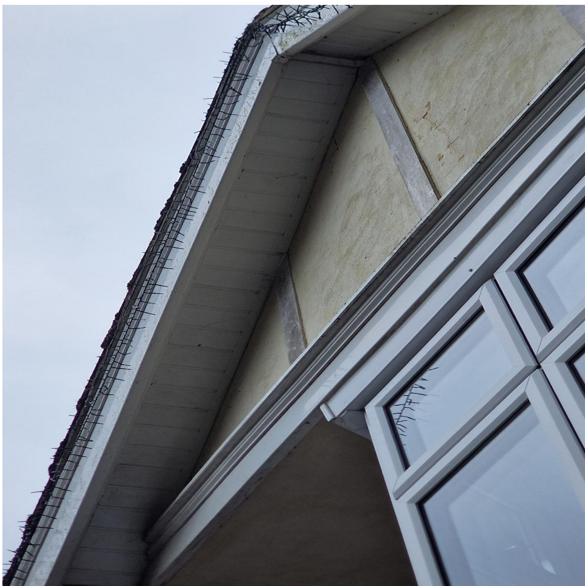
Picture 5: Showing the eaves on the front gable wall
