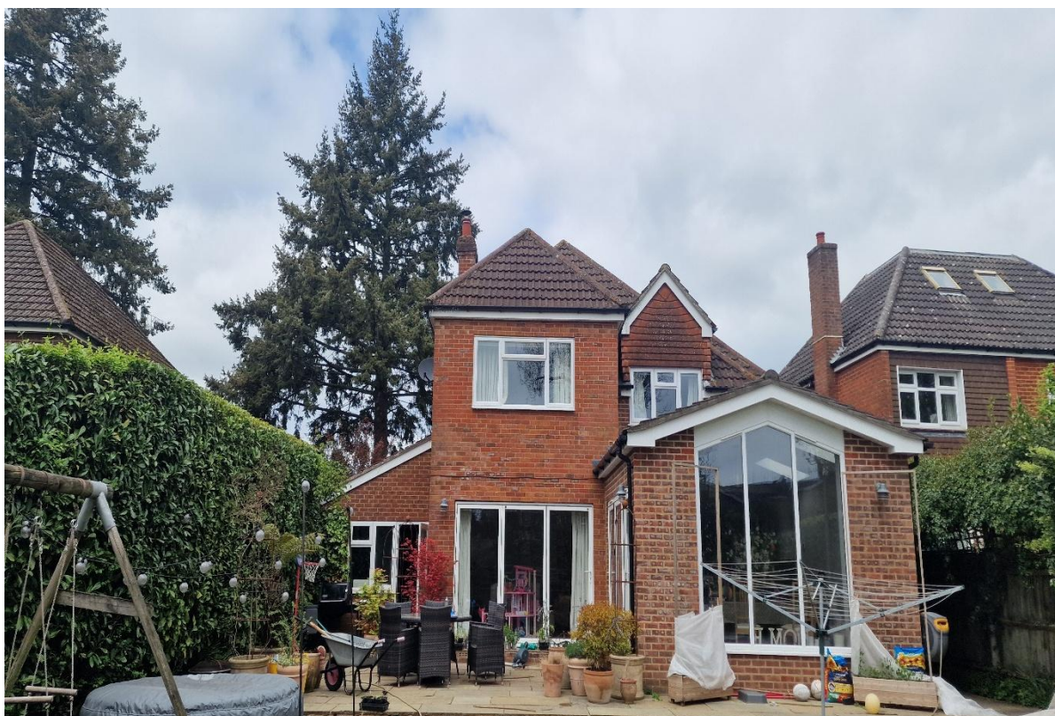
Picture 2: Showing the western elevation
