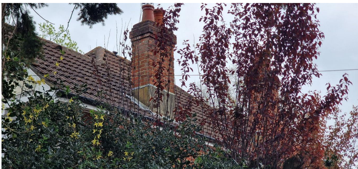
Picture 4: Showing the side elevation and flashing around chimney
