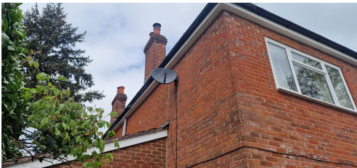
Picture 3: Showing soffit and eaves.
