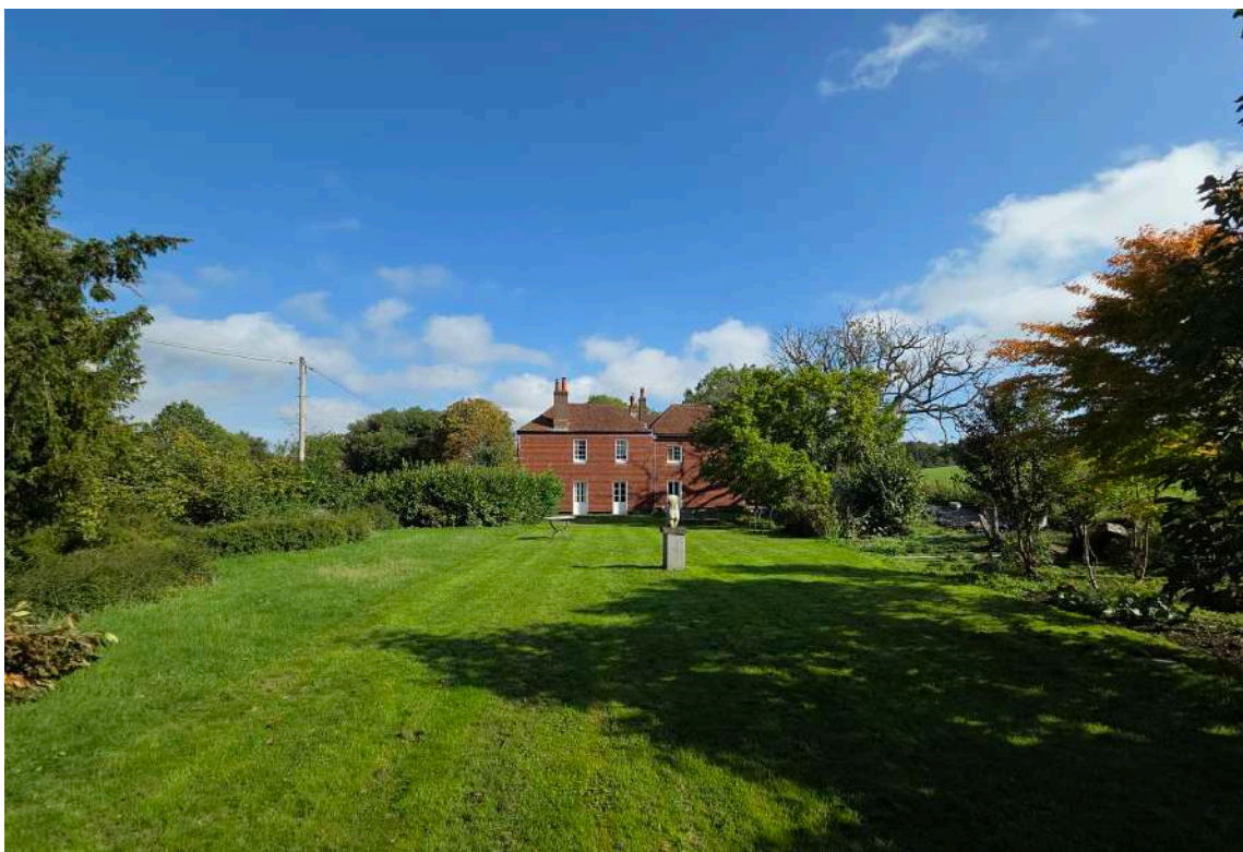
Figure 8 - Long view of South Elevation from garden
