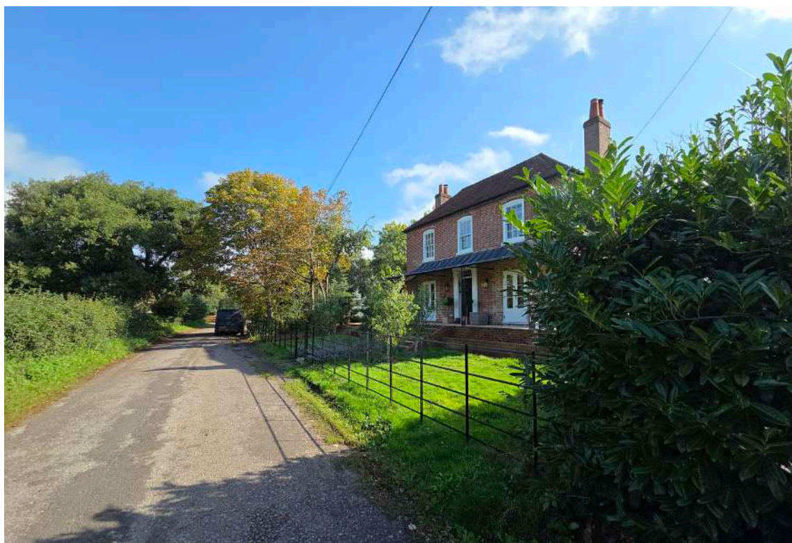
Figure 9 - Approach to Lincolns from Boyatt Lane to the South
