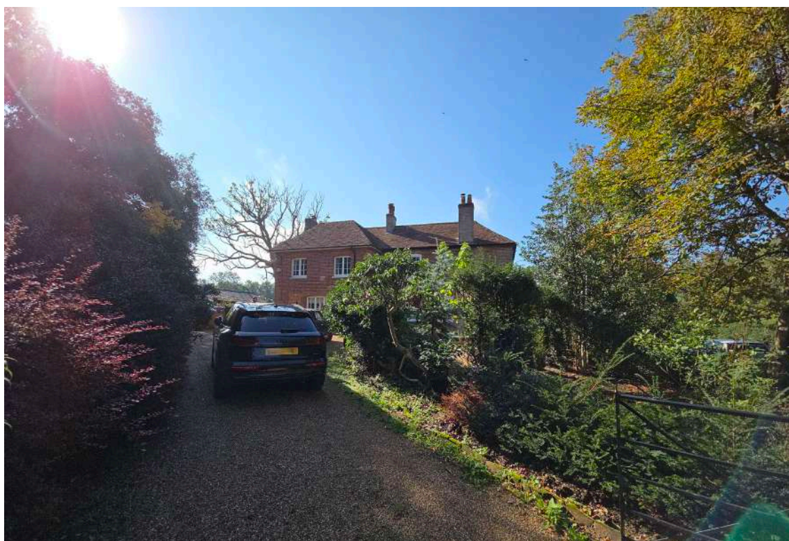
Figure 10 - Approach view of Lincolns from driveway at the intersection to Boyatt Lane
