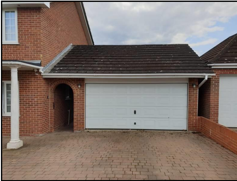
Existing Single Storey Garage (to be Removed)
