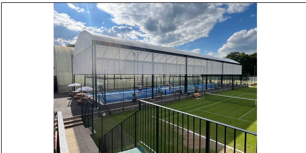
Photo 1 – Example of Modular Canopy Structure
