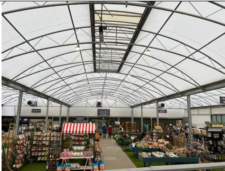
Photo 3 - White membrane roofs to Holt Garden Centre
