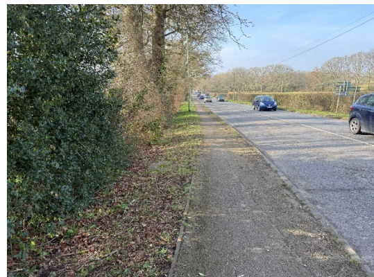
Photograph 4: Bubb Lane Shared Facility
