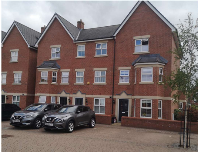
Fig 2. Existing house with parking to front (No 8 is middle property without a gable end)
