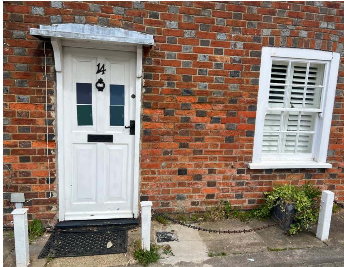
Figure 4 - No.14 Satchell Lane entrance and ground floor window.
