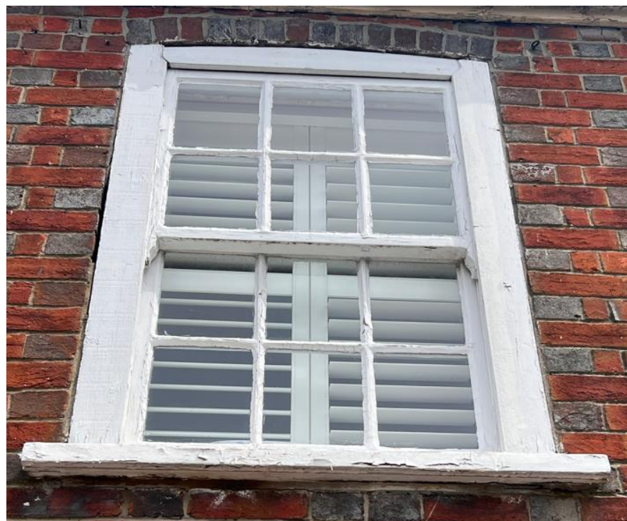
Figure 5 - No.14 Satchell Lane first floor window as existing.
