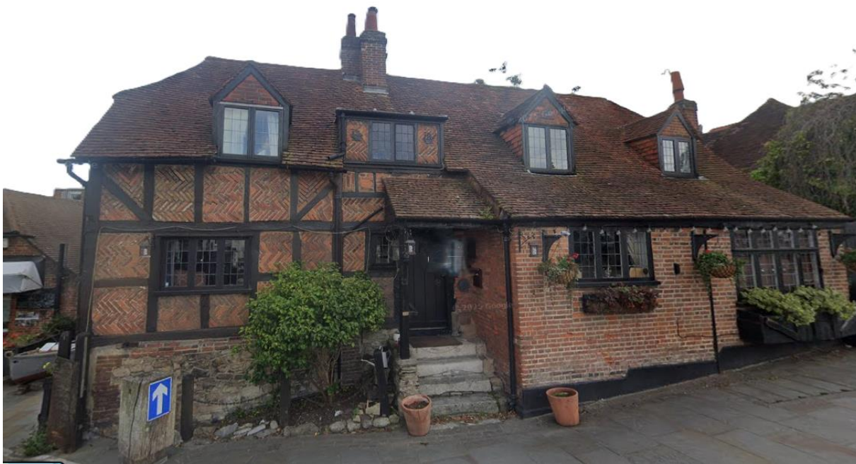
Figure 2 - C17 Grade II listed, The Old House, Hamble Square (Google Streetview)
