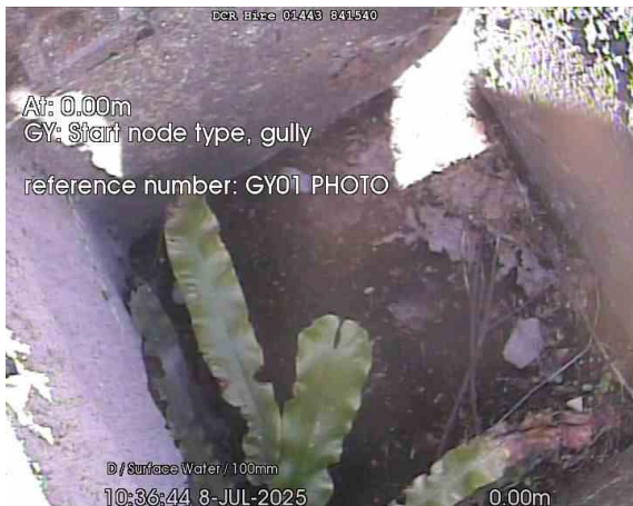
GY01 PHOTO_0-00m_103644.jpg, 00:00:00, 0.00 m Start node, gully, reference: GY01 PHOTO
