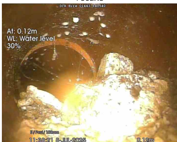
MH06 US_0-12m_113821.jpg, 00:00:04, 0.12 m Water level, 30% of the vertical dimension
