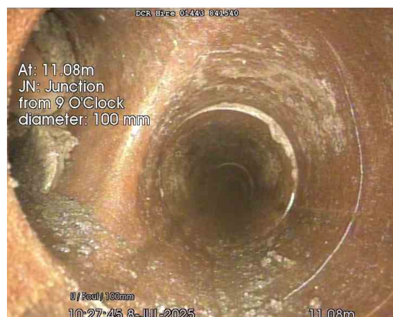
MH05 US_11-08m_102745.jpg, 00:00:39, 11.08 m Junction at 9 o'clock, 100mm dia
