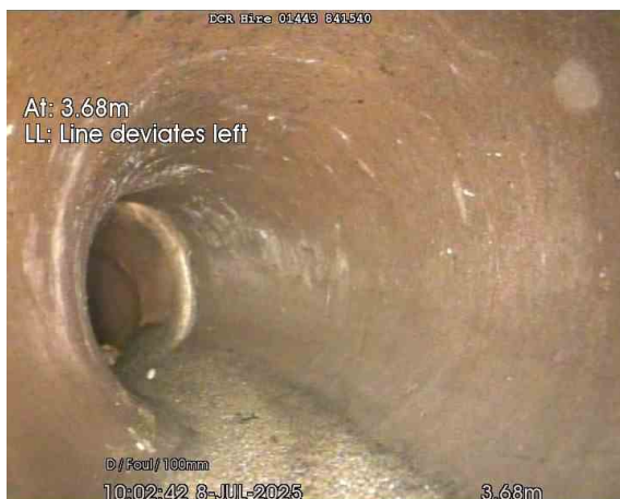
MH03 DS_3-68m_100242.jpg, 00:00:26, 3.68 m Line deviates left
