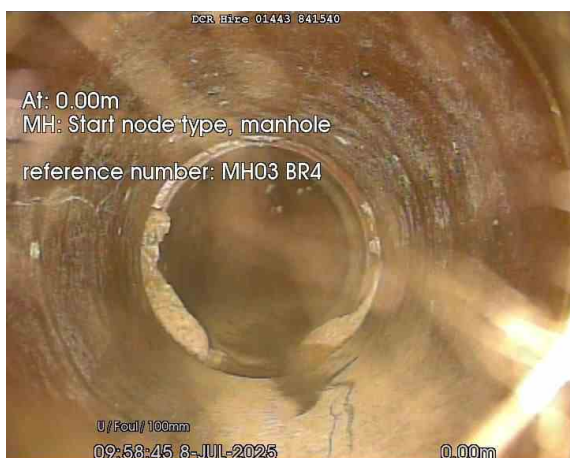
MH03 BR4_0-00m_095845.jpg, 00:00:02, 0.00 m Start node, manhole, reference: MH03 BR4
