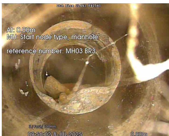
MH03 BR3_0-00m_095602.jpg, 00:00:00, 0.00 m Start node, manhole, reference: MH03 BR3
