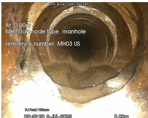
MH03 US_0-00m_094920.jpg, 00:00:02, 0.00 m Start node, manhole, reference: MH03 US
