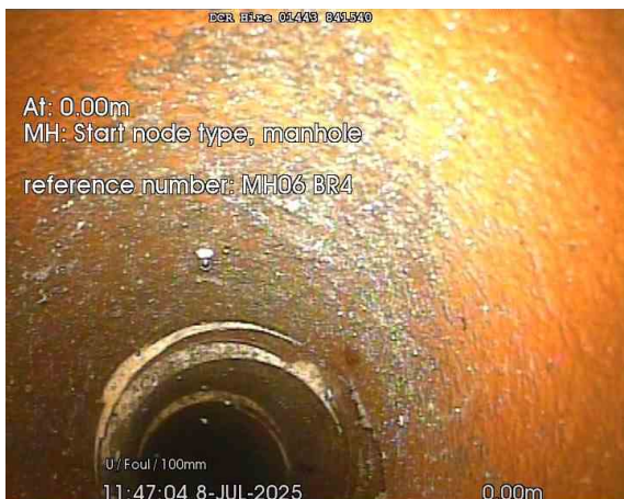
MH06 BR4_0-00m_114704.jpg, 00:00:00, 0.00 m Start node, manhole, reference: MH06 BR4
