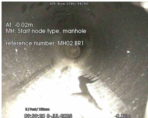
MH02 BR1_-0-02m_093920.jpg, 00:00:00, -0.02 m Start node, manhole, reference: MH02 BR1
