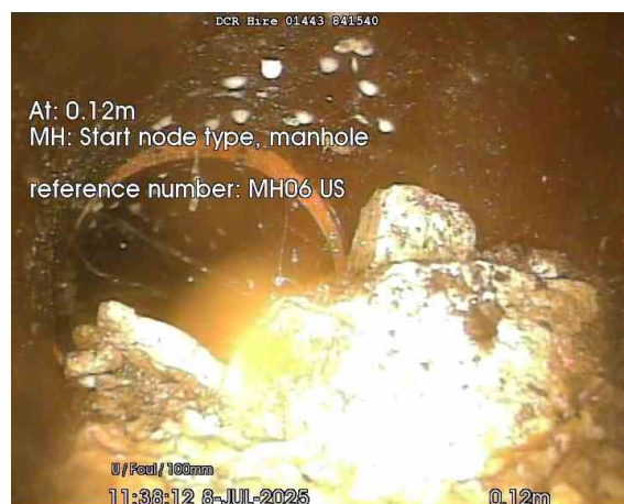
MH06 US_0-12m_113812.jpg, 00:00:02, 0.12 m Start node, manhole, reference: MH06 US
