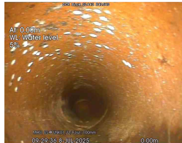
MH01 US_0-00m_092936.jpg, 00:00:02, 0.00 m Water level, 5% of the vertical dimension
