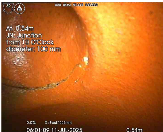
FW2301 DS_0-54m_060109.jpg, 00:00:23, 0.54 m Junction at 10 o'clock, 100mm dia
