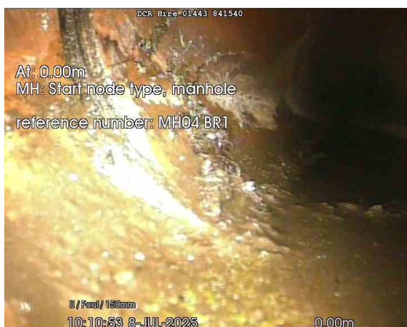
MH04 BR1_0-00m_101053.jpg, 00:00:03, 0.00 m Start node, manhole, reference: MH04 BR1
