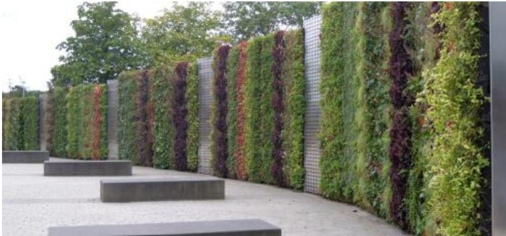
Second fix in progress. Pre-grown modules being fixed onto the wall.
