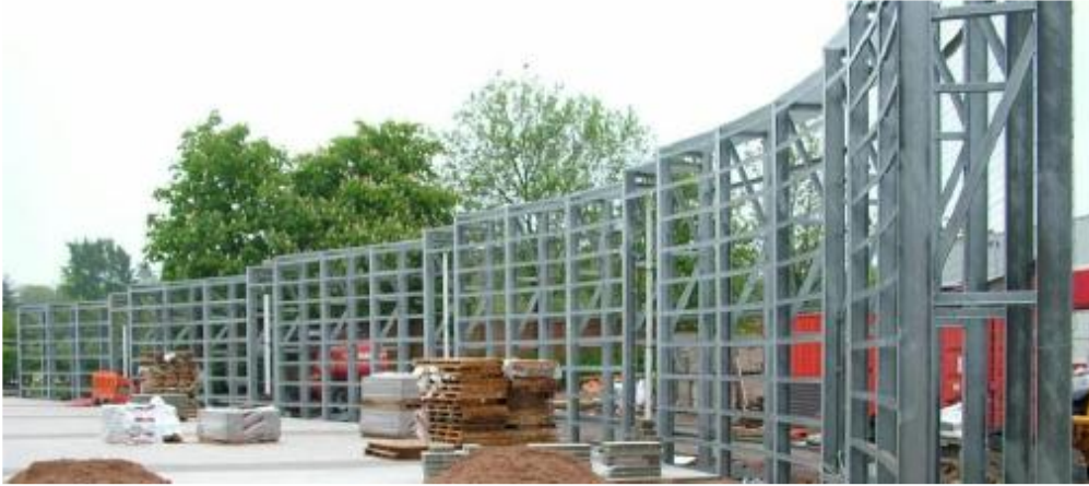
First fix in progress. Showing steel frame and hanging rails
