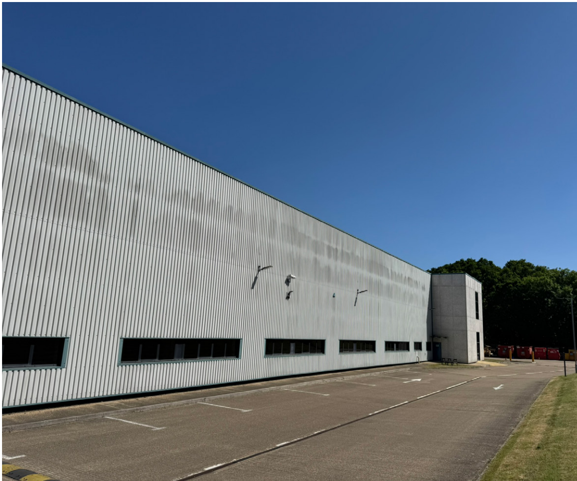
Figure 5: Northern elevation of the warehouse showing pedestrian access door and stairwell and car parking.
