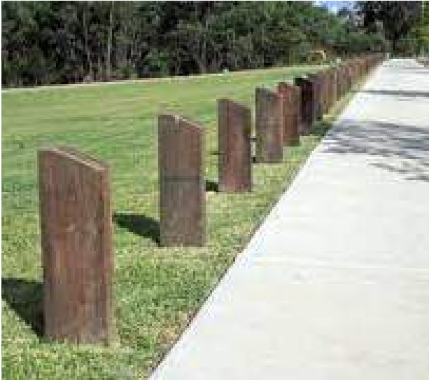
Timber posts as vehicle barriers
