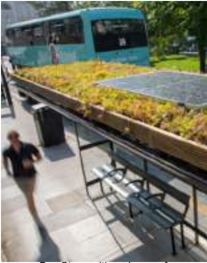
Bus Stops with sedum roofs
