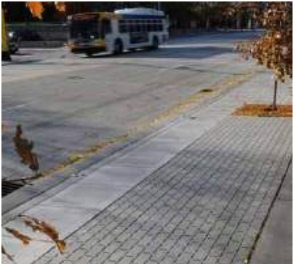
Flushed kerb edges with change of paving surfaces
