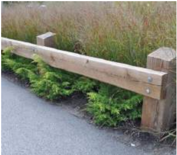
Timber knee rail fence
