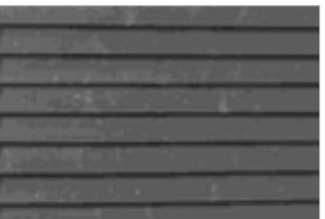
Black weatherboard boarding
