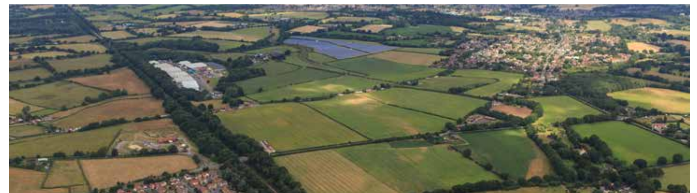
• Aerial View facing North over Bubb Lane showing larger, more regular ‘Parliamentary’ enclosure landscape
