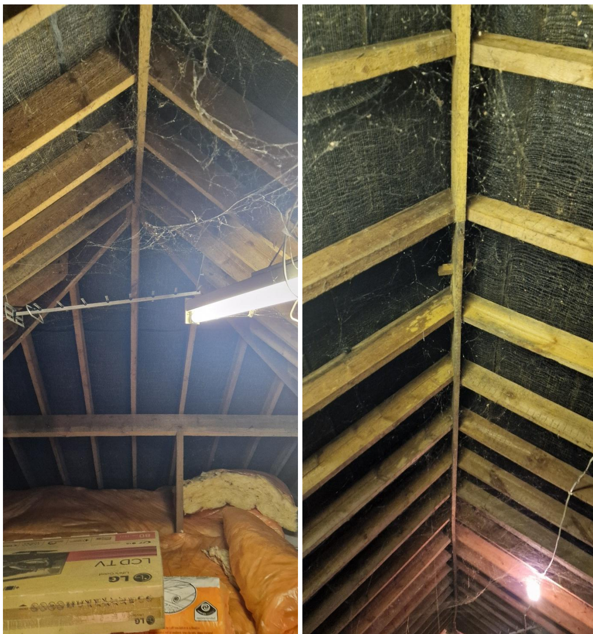
Picture 7: Showing the roof void structure
