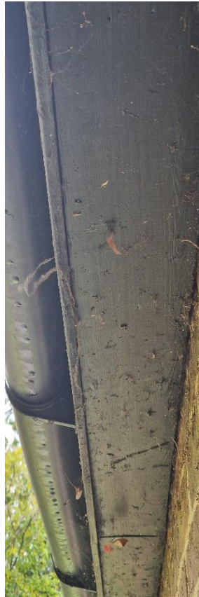
Picture 6: Showing the eaves
