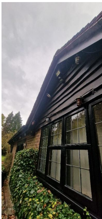
Picture 3: Showing the northern elevation where the wooden weather boarding is
