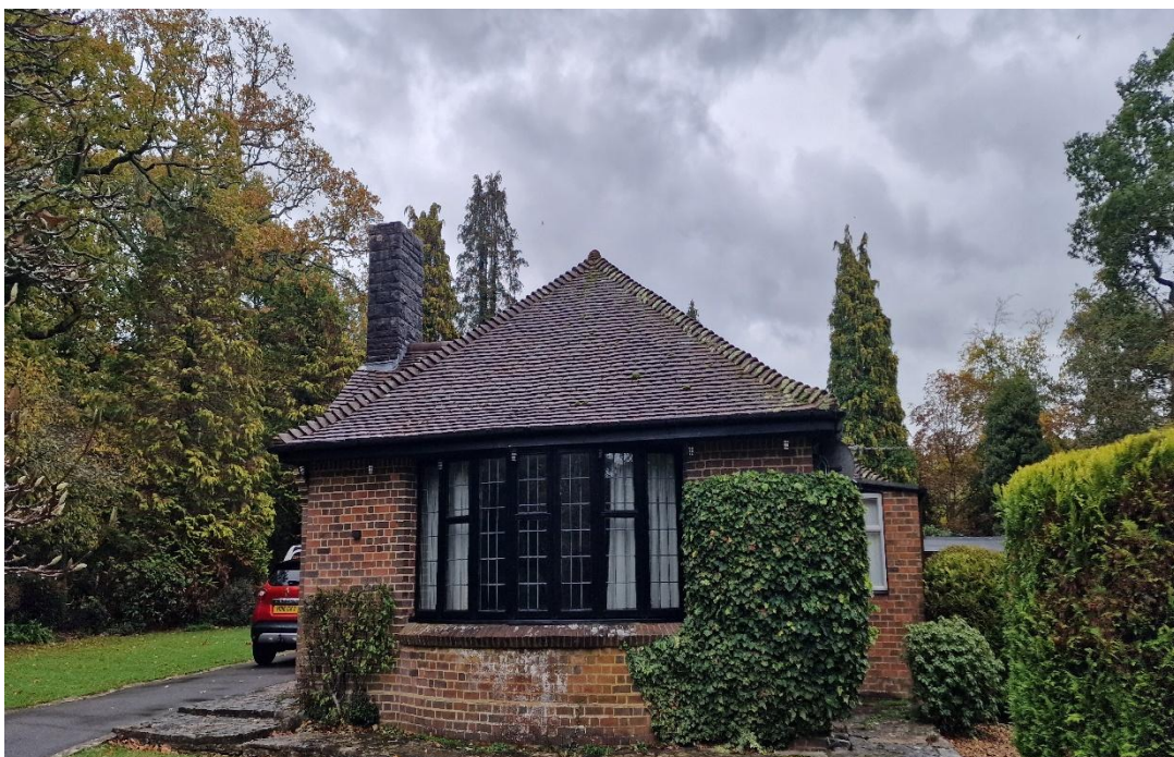
Picture 4: Showing the western elevation showing the bushes around the building
