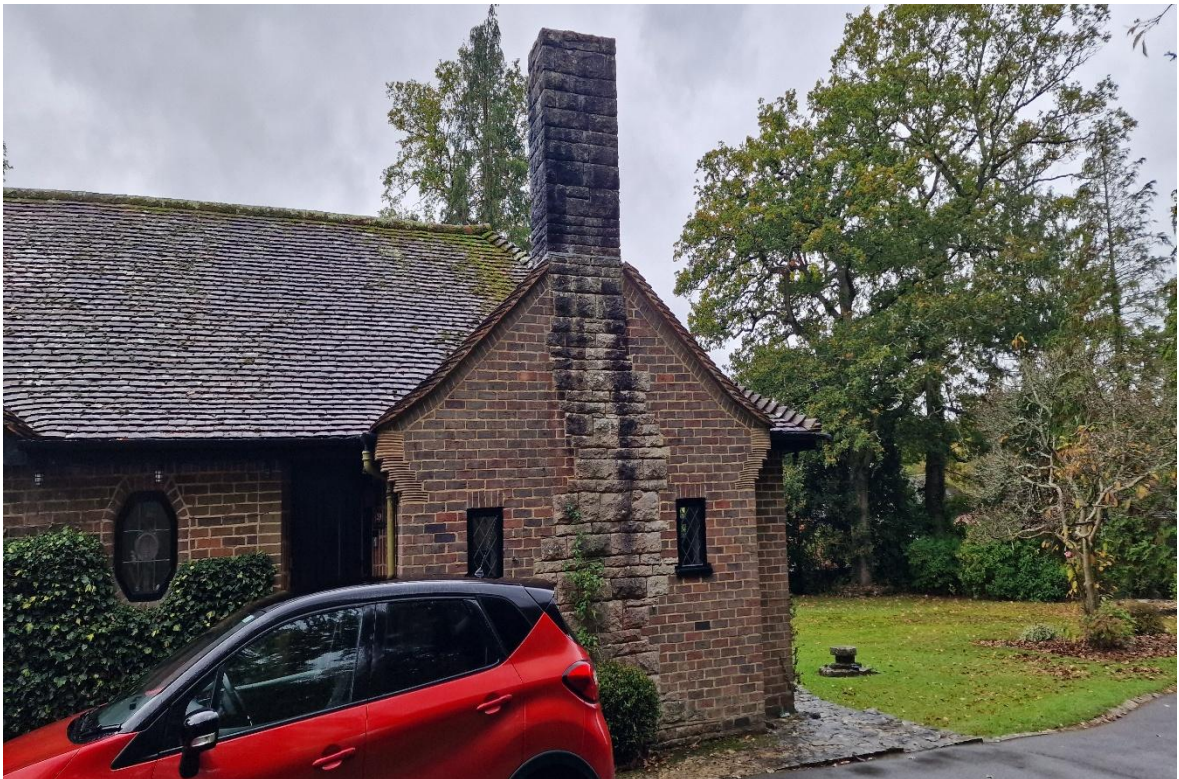
Picture 2: Showing the northern elevation
