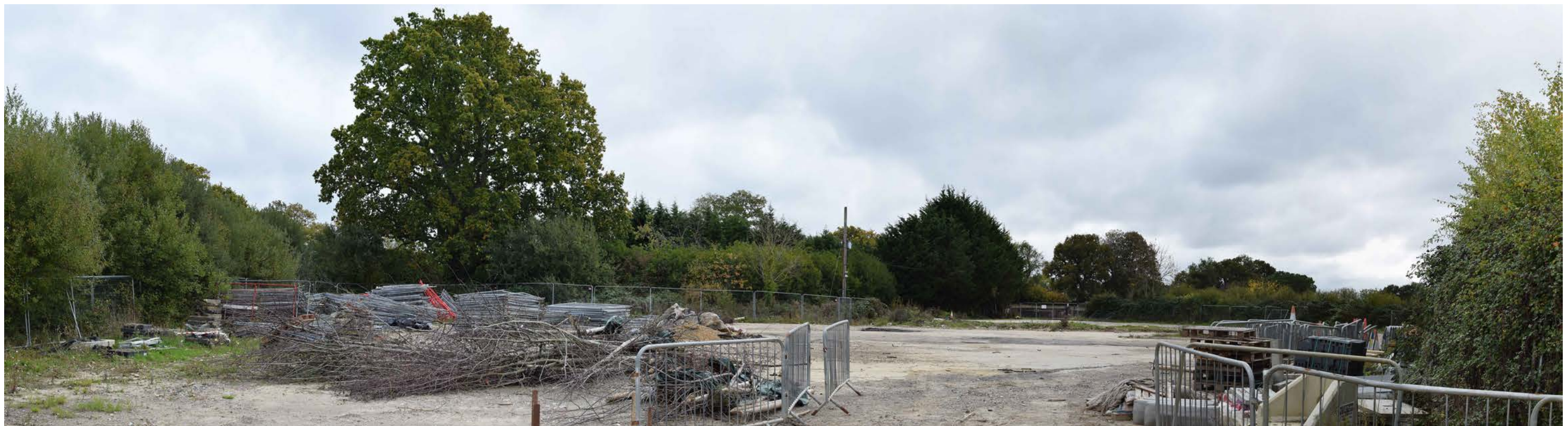
View D from location to the north of Fir Tree Lane, looking southeast across the works compound towards Fir Tree Lane
