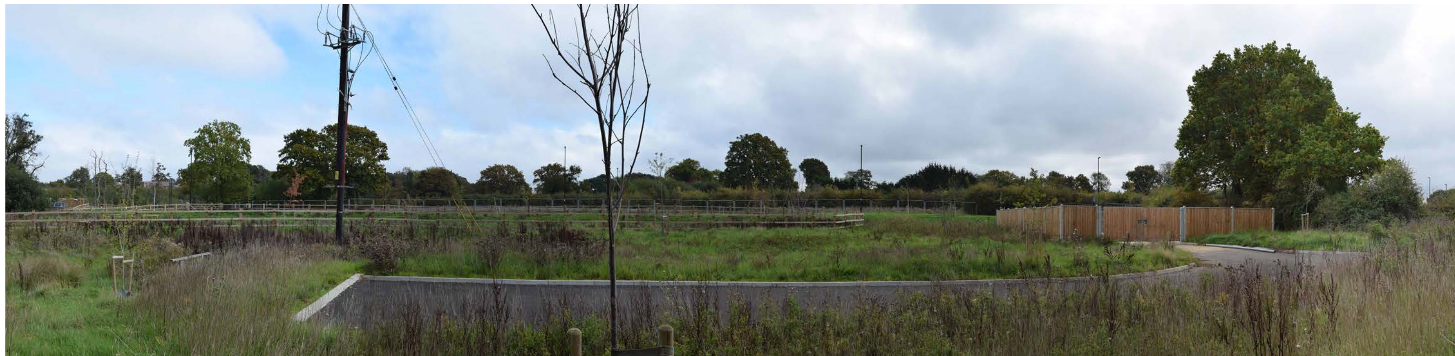
Viewpoint 11. View from footpath 085/11, looking northeast, on the western site boundary. View across attenuation basin, road and fenced pumping station in northwestern field. Topography and mature field boundary vegetation restricts views across the site to the south and east.
