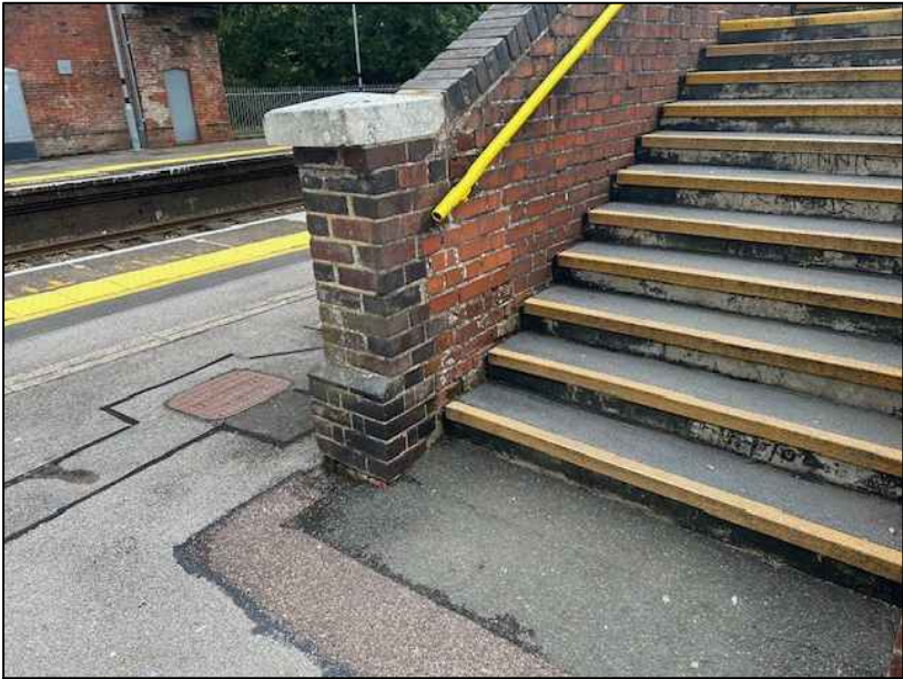
VIEW OF STAIRWAY 2 FROM PLATFORM 2 PAVEMENT TO FOORTBRIDGE
