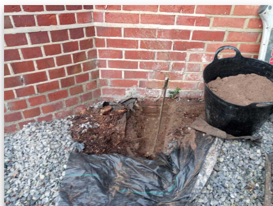
Fig 1.2: Trial Hole 1 Footing
