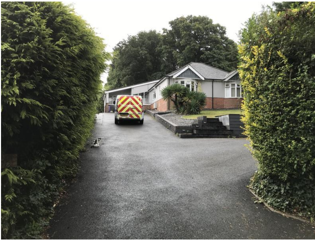
Photo 3 - Sloping site front
