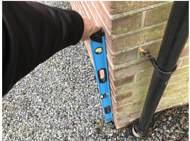
Photo 25 - Left elevation plumb
