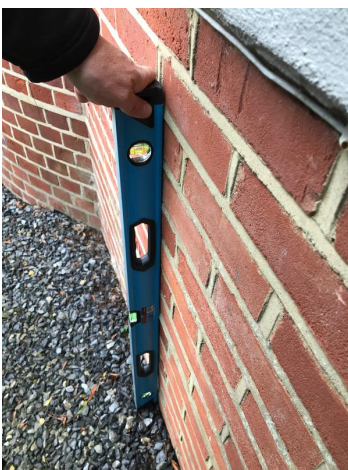
Photo 26 - Front elevation remains plumb
