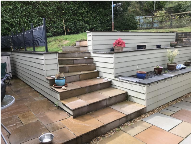
Photo 7 - Stepped retaining wall rear
