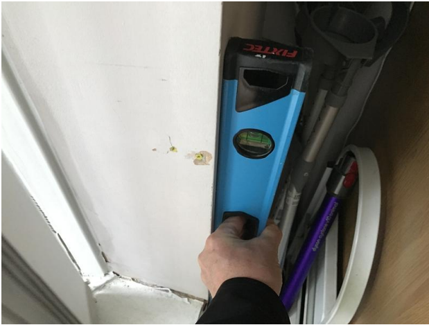
Photo 31 - Front elevation plumb
