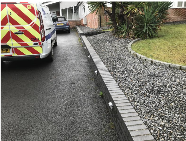
Photo 5 - Retaining wall front
