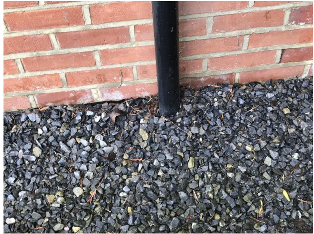
Photo 14 - Down pipe front elevation
