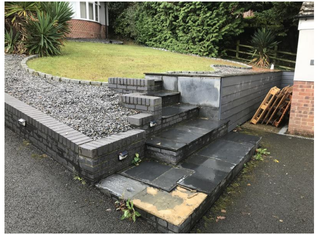
Photo 4 - Retaining wall front
