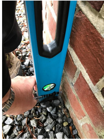
Photo 23 - Rotation 10 mm over 1 metre height
