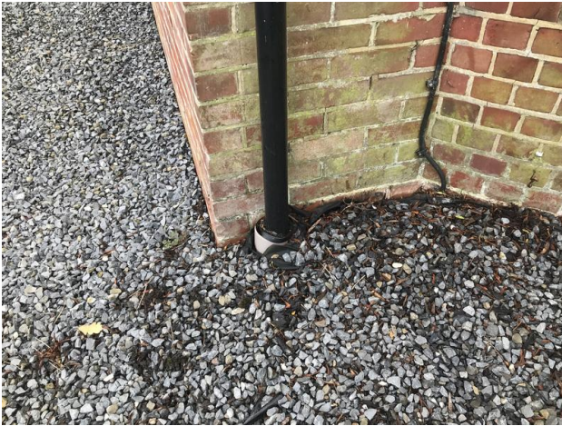
Photo 13 - Downpipe gully FLC
