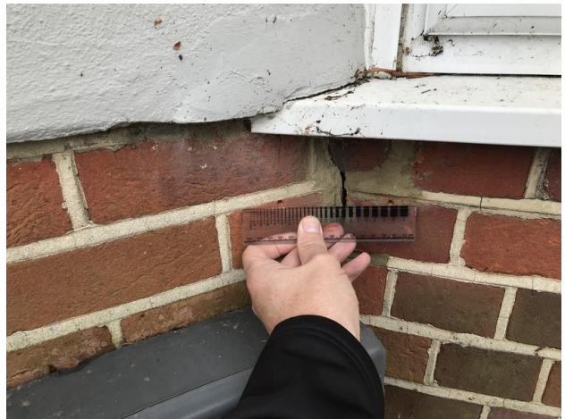
Photo 21 - Joint width 3.5 mm
