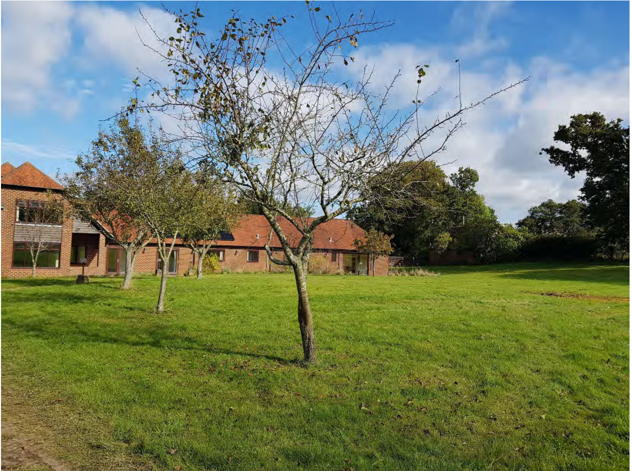
Plate 21 – View north east showing Victoria House
