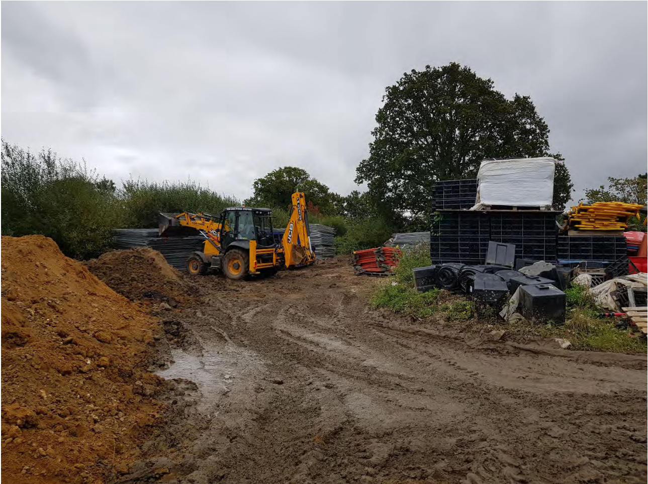
Plate 16 - Photograph showing the site compound area
