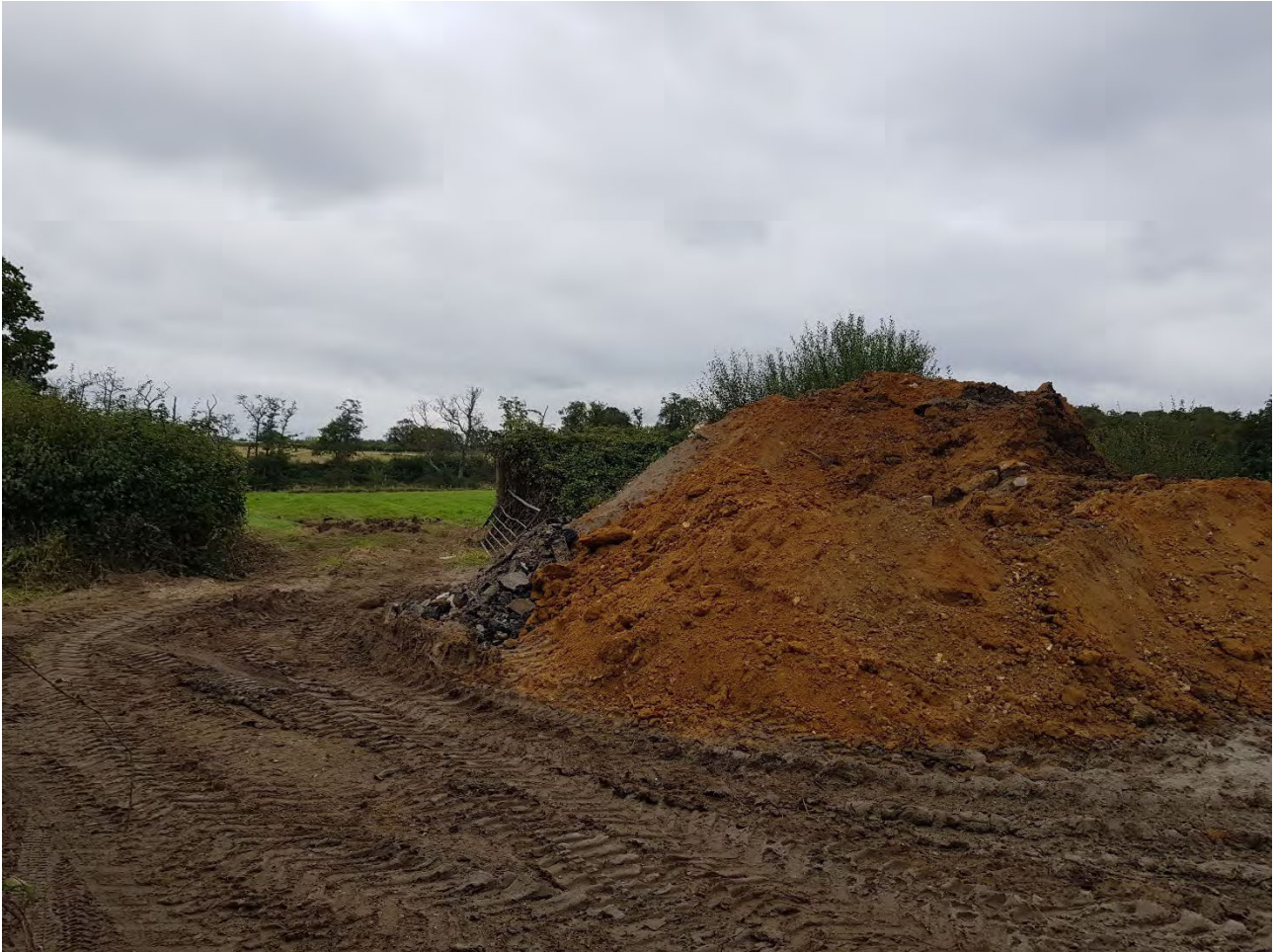
Plate 15 - Photograph showing material storage in the site compound area
