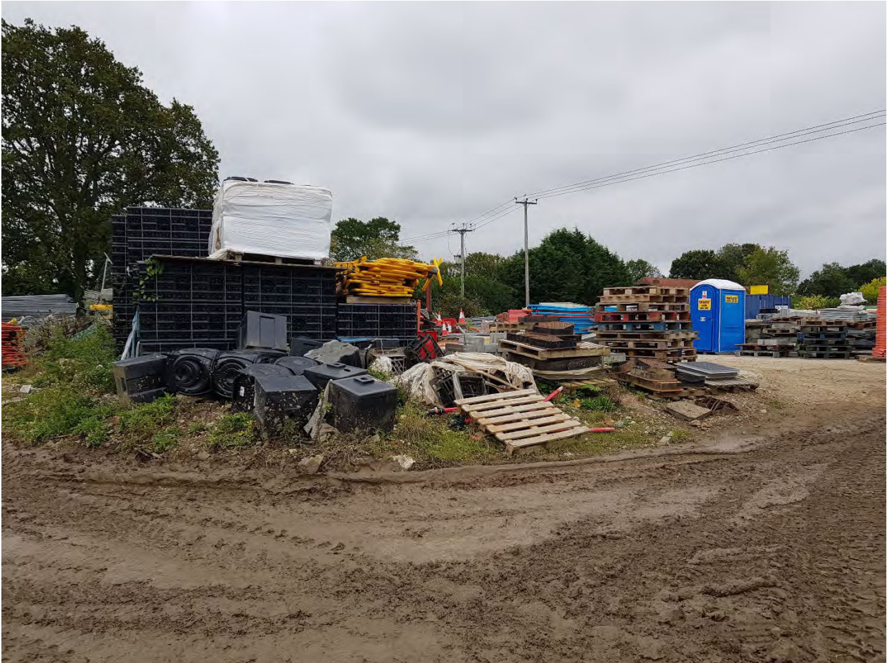
Plate 13 - Photograph showing material storage in the site compound area
