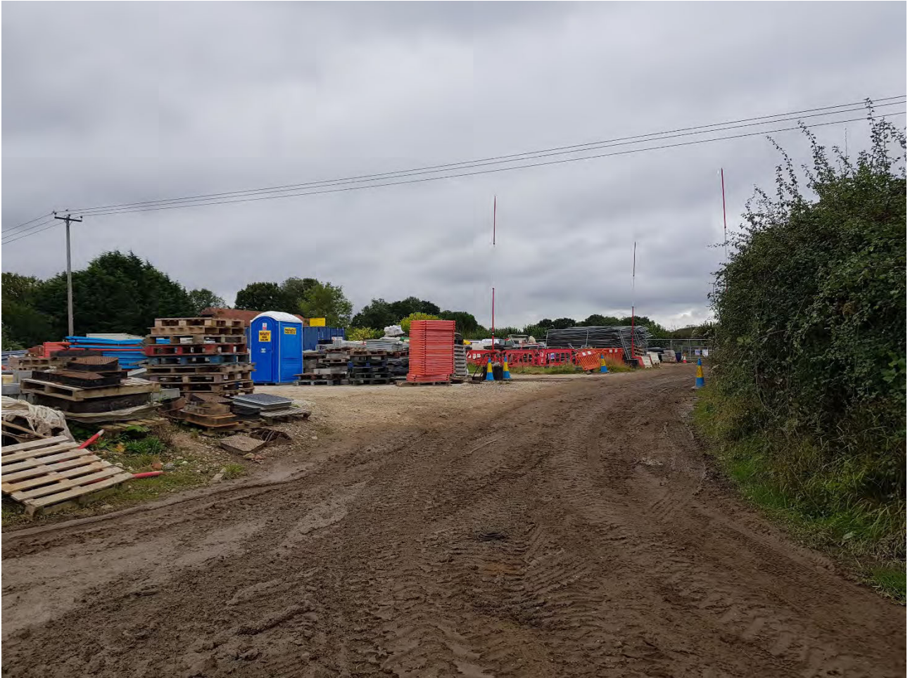
Plate 14 - Photograph showing the site compound area
