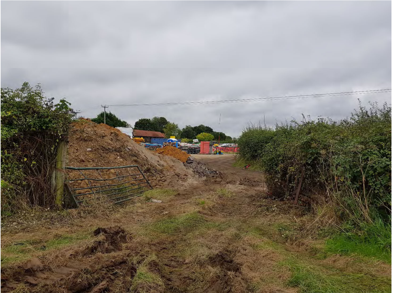
Plate 10 – View south of access from site compound to northern field
