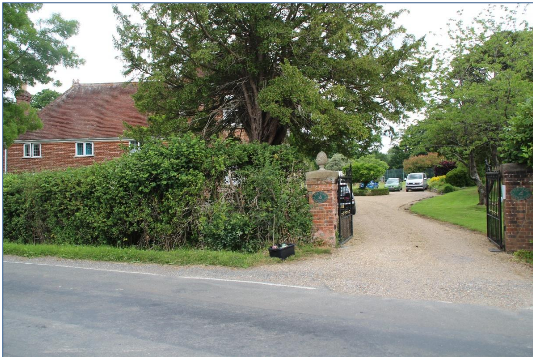
Photo 2 Fir Tree Farmhouse seen from Fir Tree Lane
