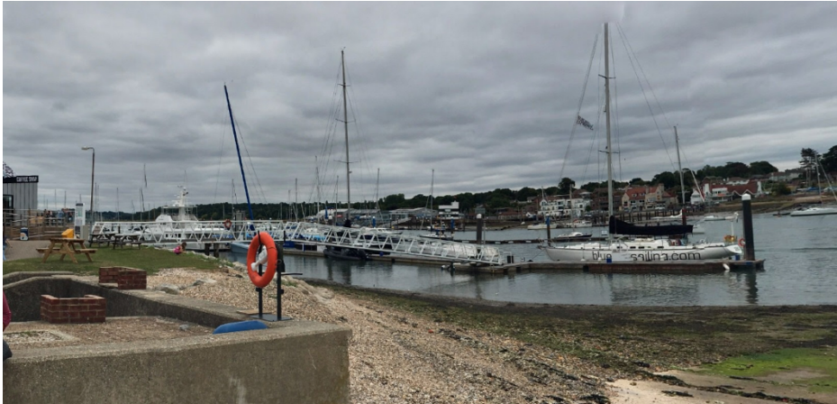
Figure 2: Existing Bridge to be Replaced
