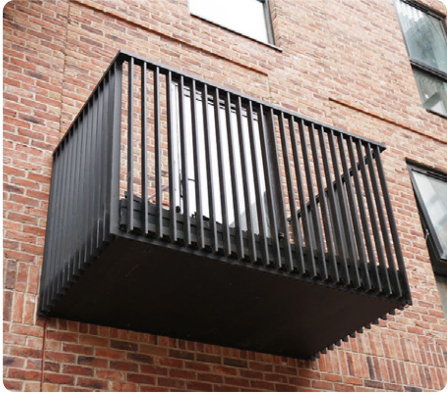
Black galvanised steel balcony
