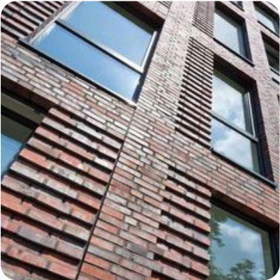
Brickwork integration with fenestration to create depth and rhythm within facade
