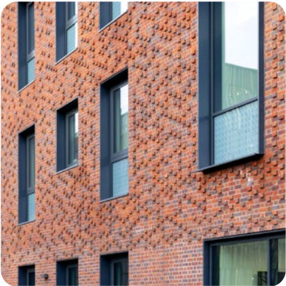
Expressed aluminium frames in some location creates playful facade and works as the antithesis element of the 'punch in' entrance
