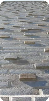
Special brick options bringing interest and definition to elevation, subtle use of different mortar colour breakup extensive facades
