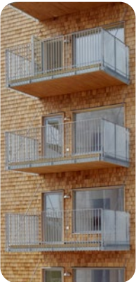
Steel frame balconies with vertical balustrades and framed in steel columns
