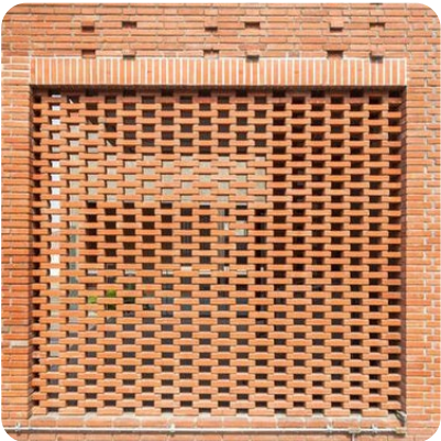
Hit and miss brickwork to allow for ventilation and natural light in cycle and refuse stores
