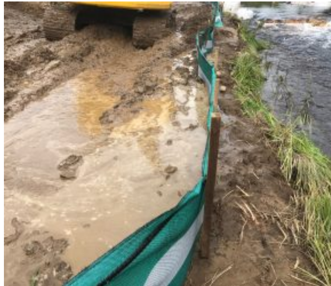
Figure 9 Example of Terrastop Premium on a working site
