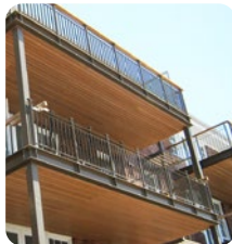
Dark steel frame balconies with timber soffits and vertical balustrades
