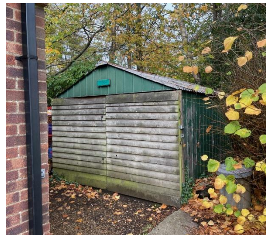
The outbuilding located adjacent to our Hall
